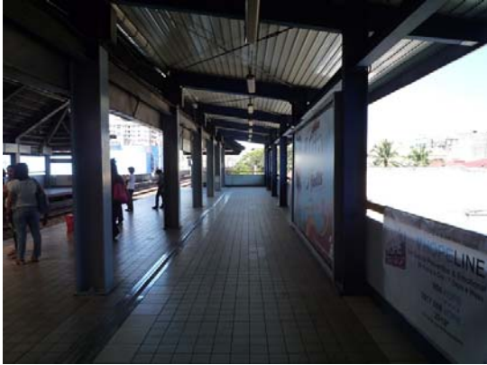
Expansion of Platform (EDSA station)
