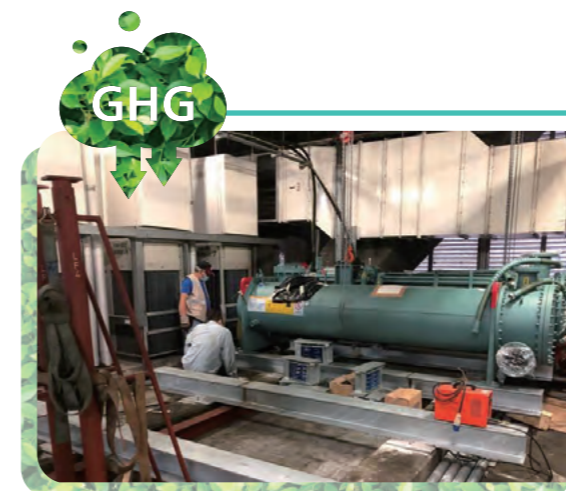
Replacement of chiller at Cheung Kong Center
