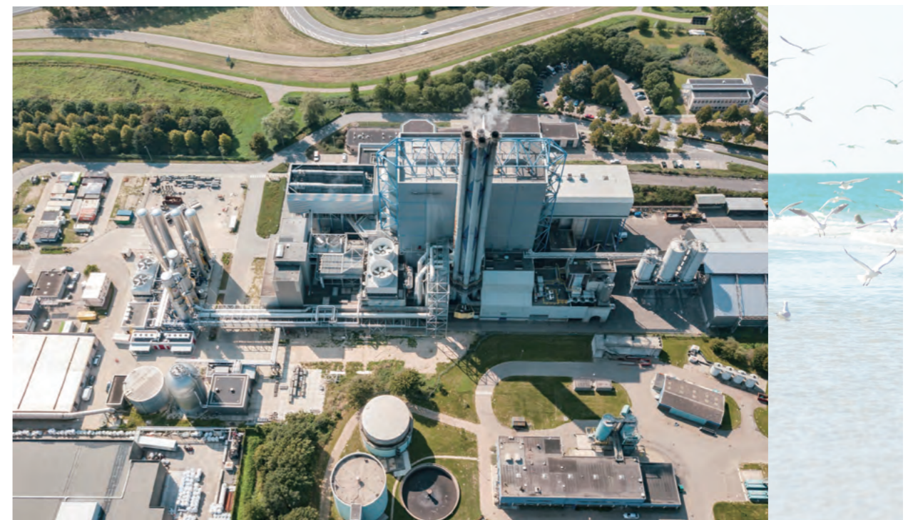
AVR's Waste-to-Energy Plant in Duiven
