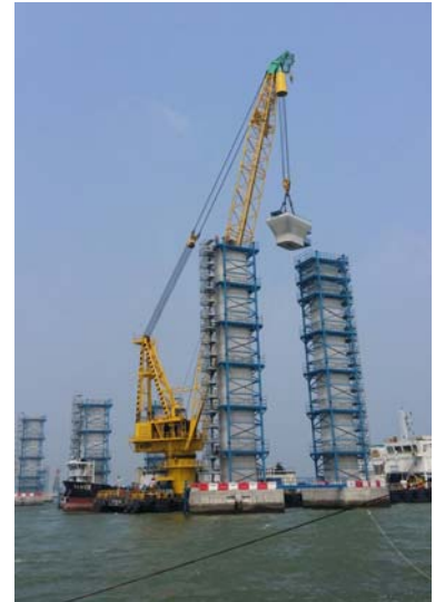
Figure 9-1- Column Erection
