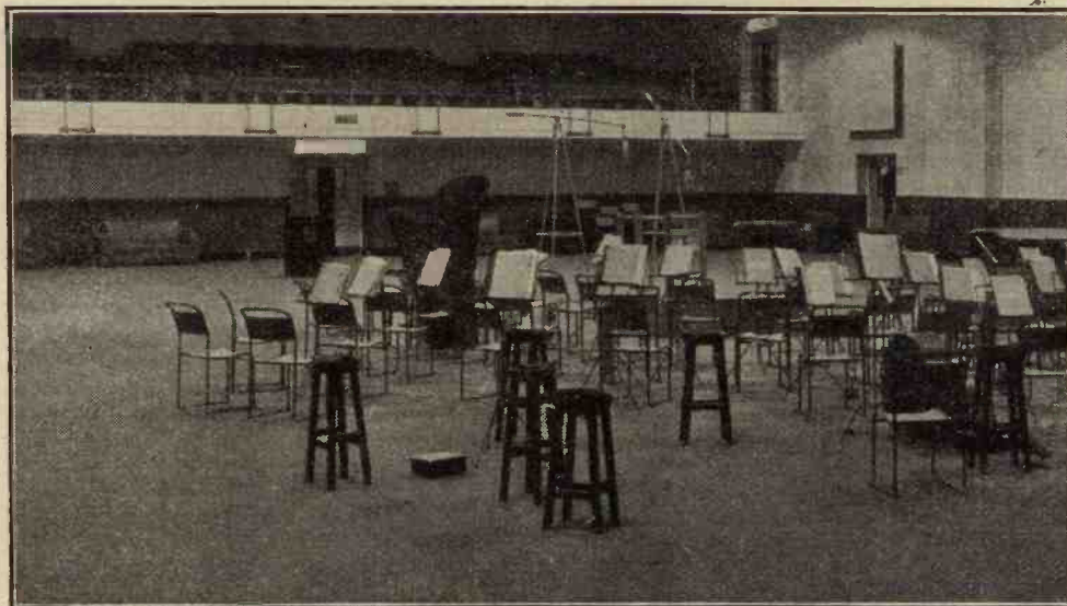
BRITAIN'S BIGGEST BROADCASTING STUDIO. The refurbished skating rink at Delaware Road, Maida Vale, which is now in regular use by the B.B.C. The floor area is 110 x 72 feet and the volume is 220,000 cubic feet.
