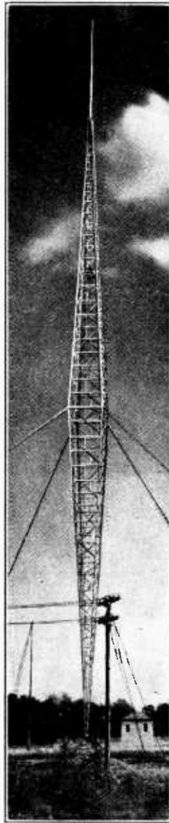
Programmes from the Columbia Key station, WABC, New York, are sent out in medium and short waves. The photograph shows the adjustable short-wave aerial.
