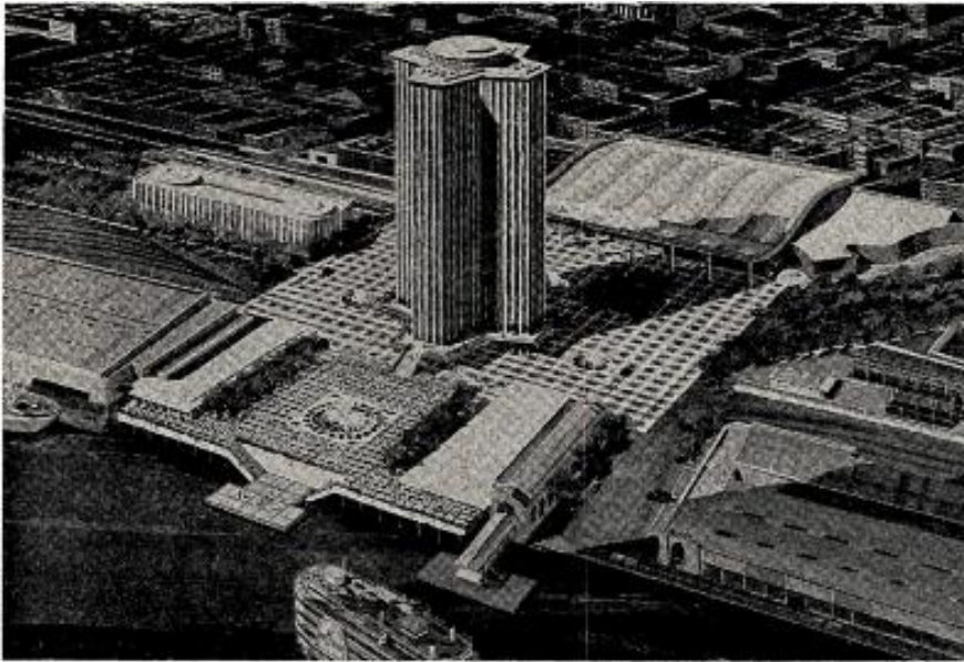
The new $40 million International Trade Mart Building in New Orleans is one of the busy city's most ambitious
