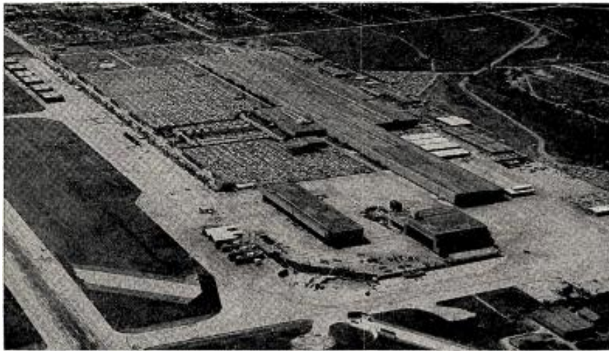
The General Dynamics Corp. Convair division plant at Ft. Worth includes a 4,000 foot long assembly building. The reservation covers 607 acres.
