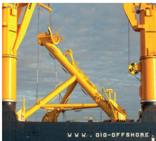
The substructure of the HS1000 tidal turbine on its way from the Arnish Yard near Stornoway, where it was constructed, to Orkney.
