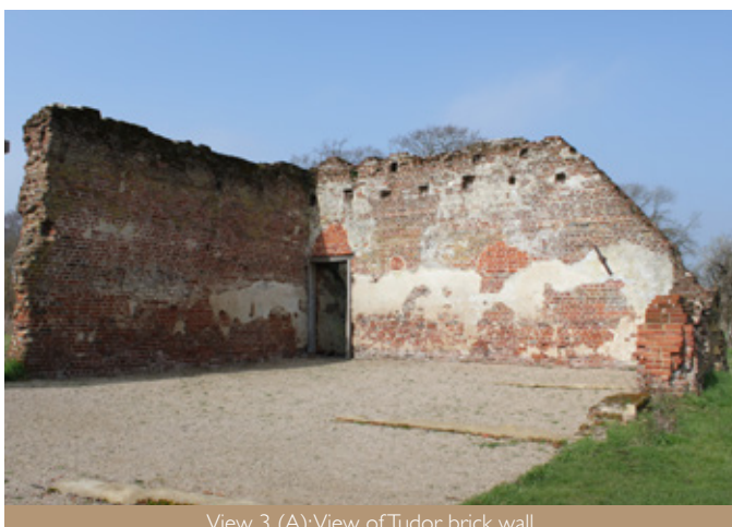
View 3 (A): View of Tudor brick wall
