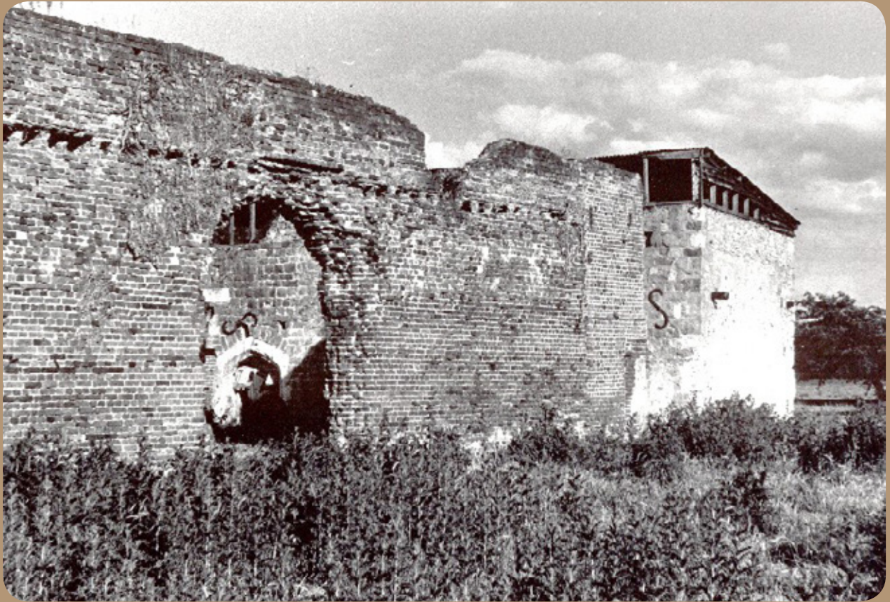
View of Palace from north west. c.1985. Note intact monopitch roof to vault and brick arch. (Reproduced by permission of Phillip Moll).
