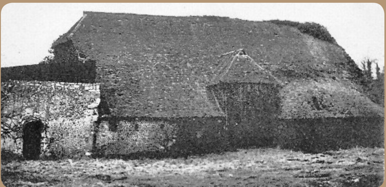
View of barn and vaulted room from north west, believed to be c.1905. Note intact roof to barn building and monopitch roof to vault. (Reproduced by permission of Phillip Moll).
