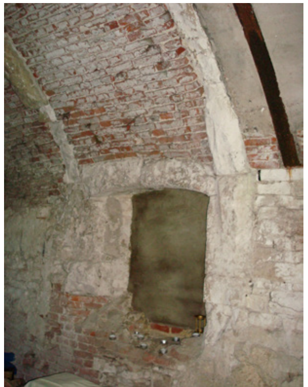
Internal view of vaulted structure
