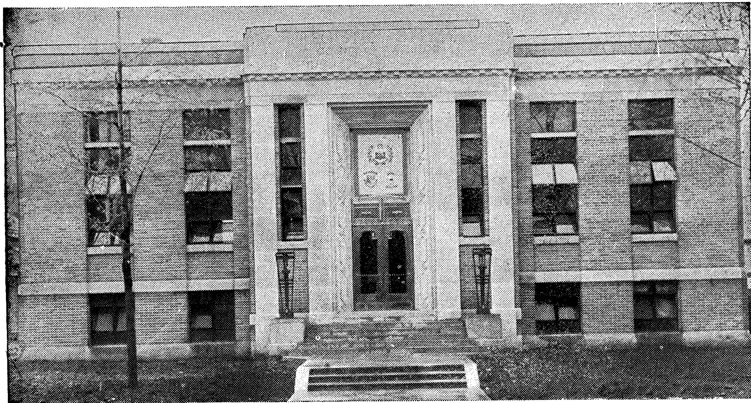
REGISTRY OFFICE, WATERLOO COUNTY ERECTED 1939
