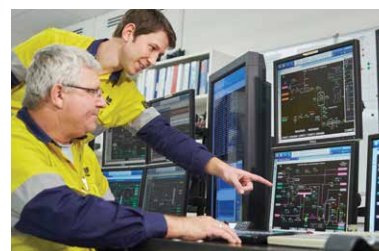
From left, Jeff Embleton and Greg Luyt in the ammonium nitrate control room in CSBP's Kwinana works, in Western Australia.
