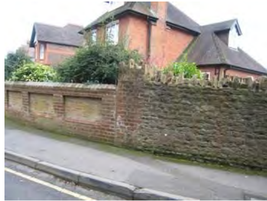
Original style Victorian brick and stone walls
