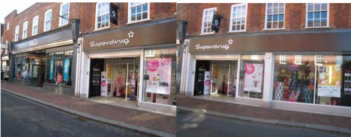
The shop on the left has divided the frontage with wooden painted windows and risers which fits with the street scene
