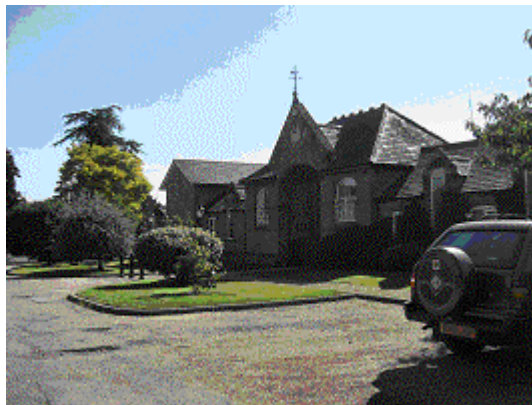
Part of Bramley Park Court. Added to the CA in 1990.
