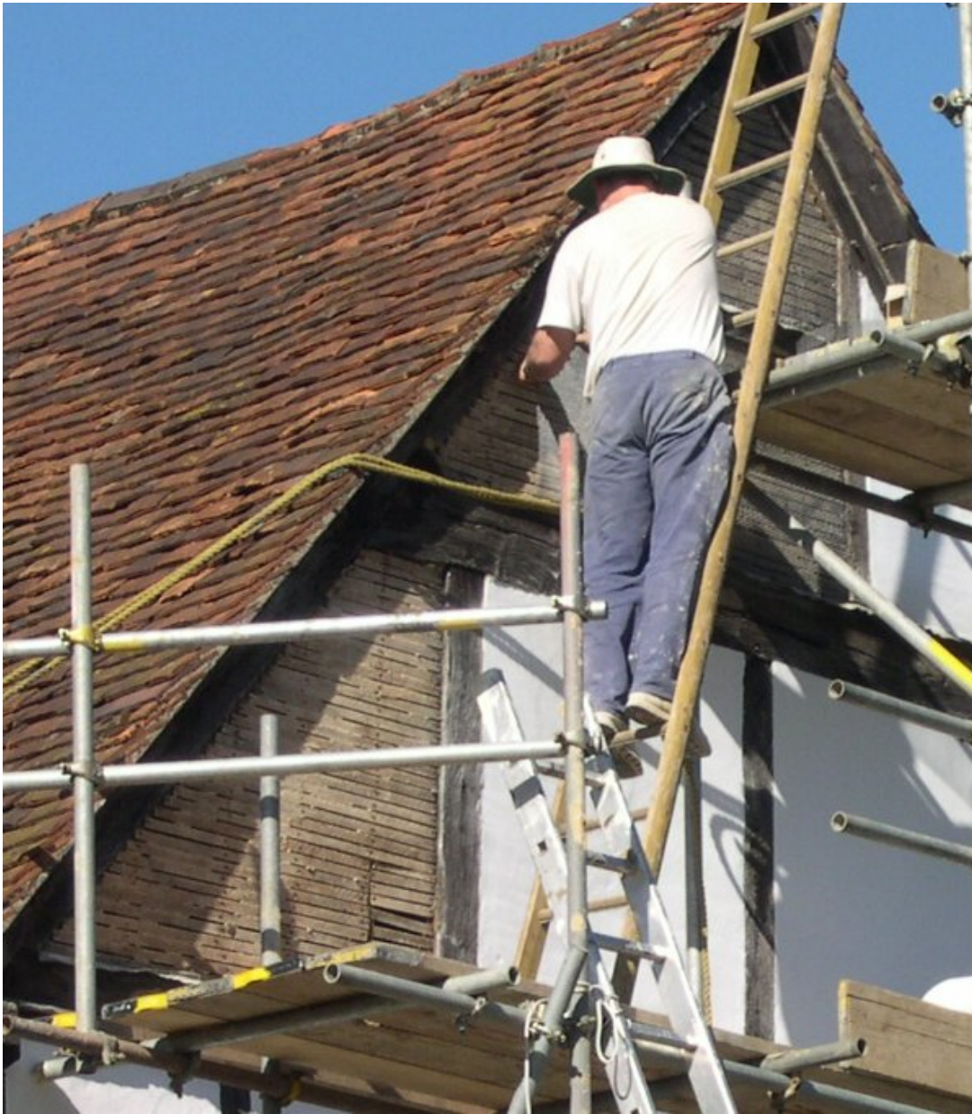
Working on a Listed Building in Horsham Road
