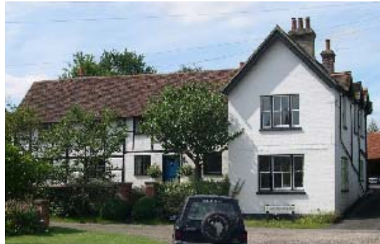
Left above: East Manor Left: Summerpool Cottage Right: Saddlers
