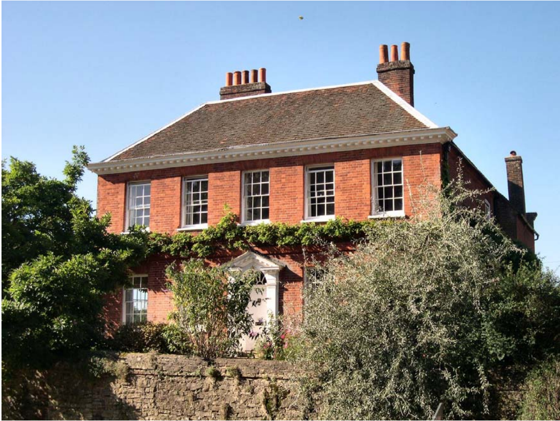
Summerpool House, High Street.
