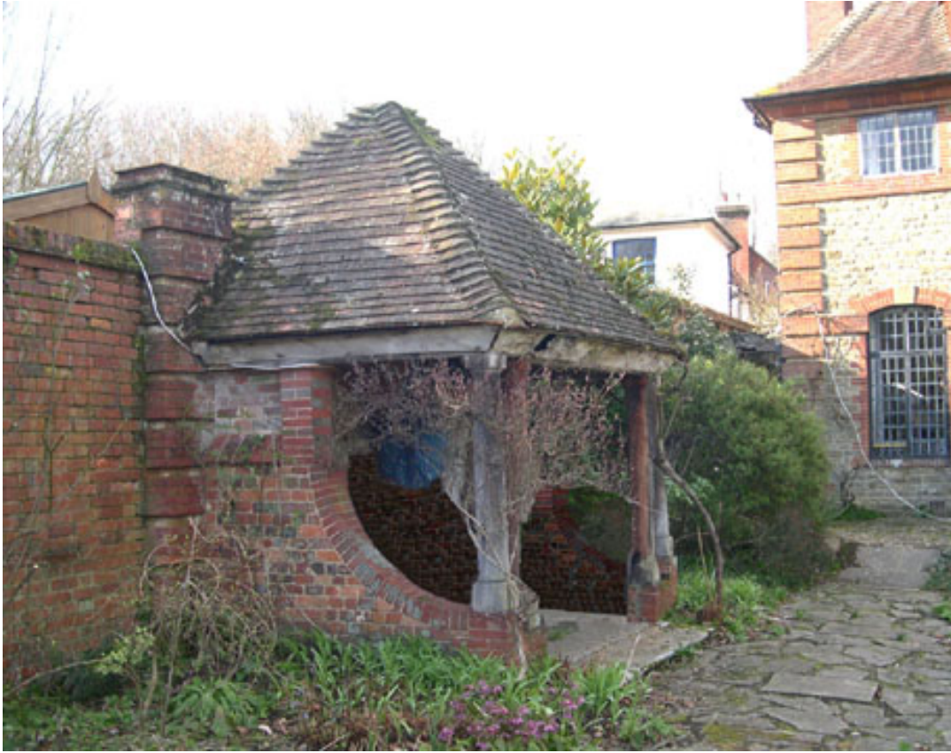
The Summerhouse at Millmead, Snowdenham Lane
