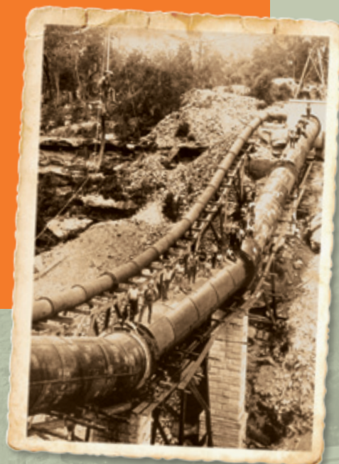
The Hudsons' Temporary Scheme is shown here as the smaller pipe running alongside the large, permanent Upper Nepean Scheme pipeline. In 1888 the temporary infrastructure was dismantled.
