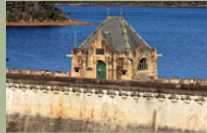
Cataract Dam, built by 1907 to expand the Upper Nepean Scheme.
