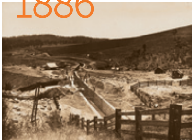
Construction of the Upper Canal in 1886. The primitive huts which housed the workers can be seen on the far right of the photograph.
