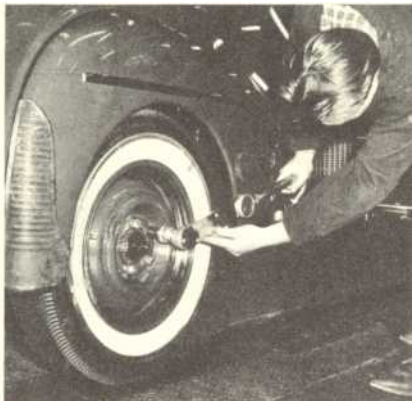
Final inspection of all functions: checking wheel nuts with torque-wrench.
