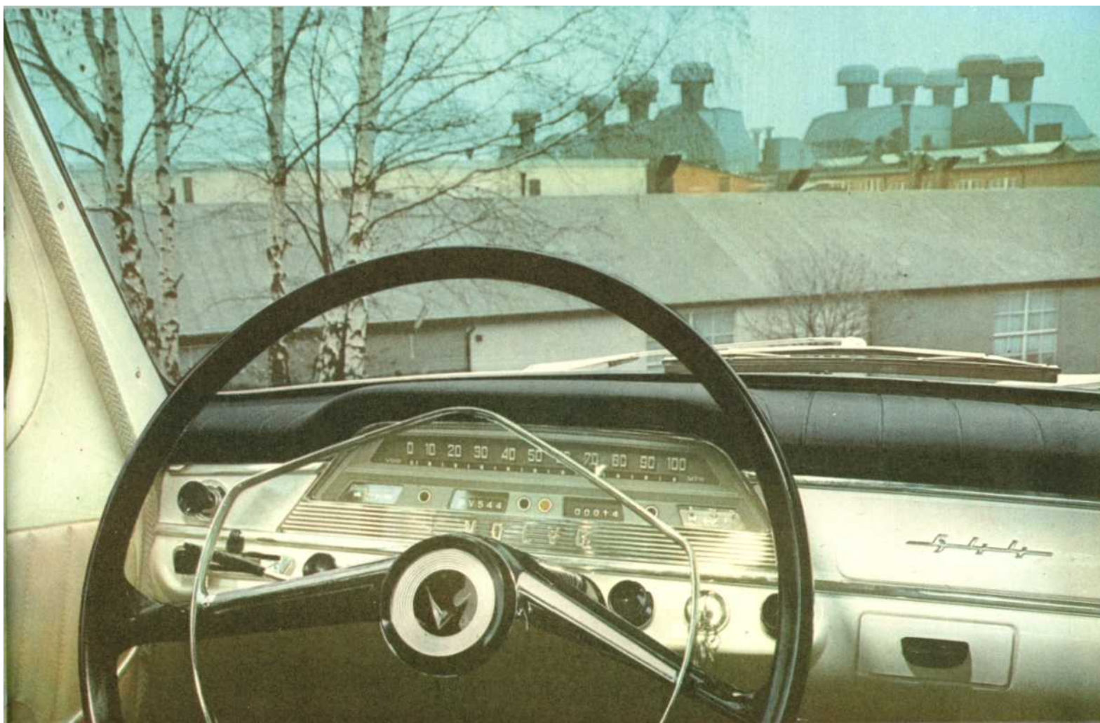
A first glimpse of the Volvo plant. Those strange-looking "mushrooms" help ventilate the spray booths in the painting department.
