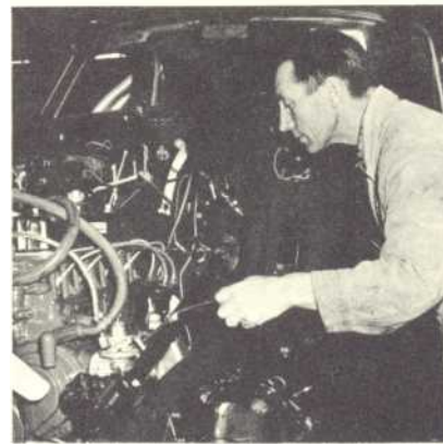
Inspection of brake cylinder for fluid, inspection of steering, motor and other components.
