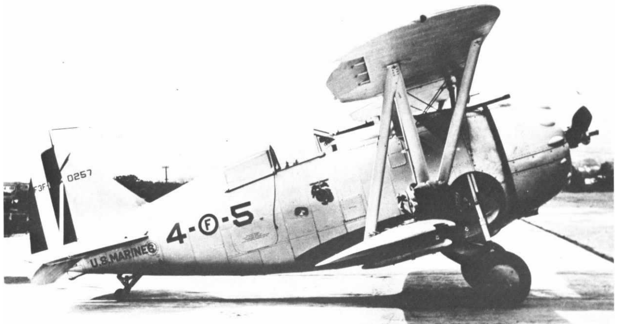
An F3F-1 of VF-AM. This was the first Marine fighter with retractable landing gear. (Photo from Museums Branch Activities, Quantico).
