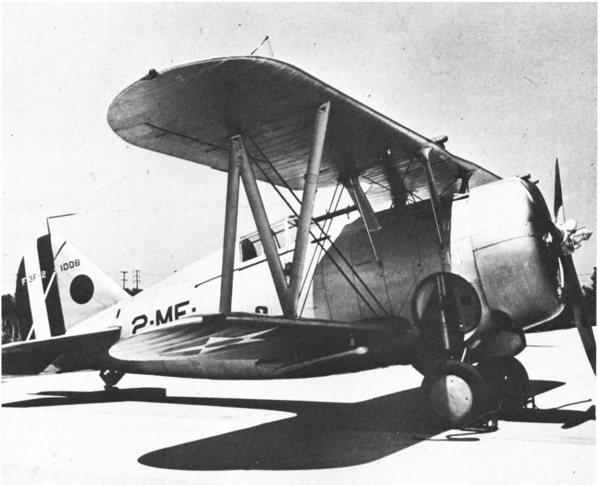
Last of the Grumman biplanes, an F3F-2 with closed cockpit and three-blade propeller in 1938. (Marine Corps Photo 525776).
