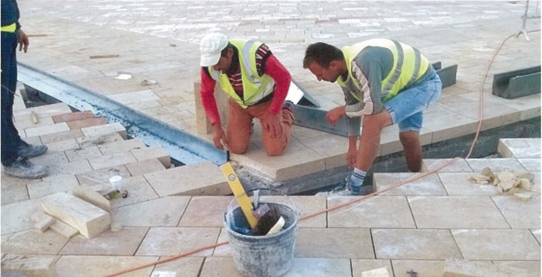
Paving and installation of rain water collection system. GHRC
