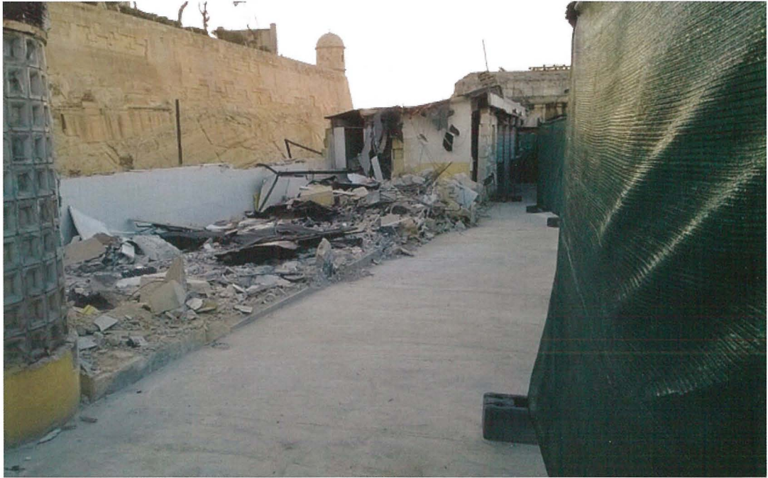
Demolition works of old and derelict kiosks. GHRC
