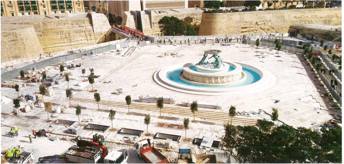
Final phases of works at Triton Square. GHRC
