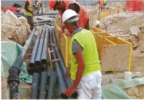
Installation of PVC pipes for services. GHRC.
