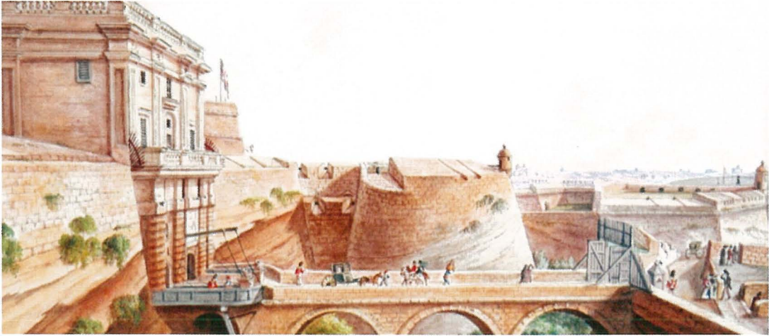
Charles F. Von Brocktorff, 1835c, Porta San Giorgio constructed in 1633 after the design of Tumas Dingli.
