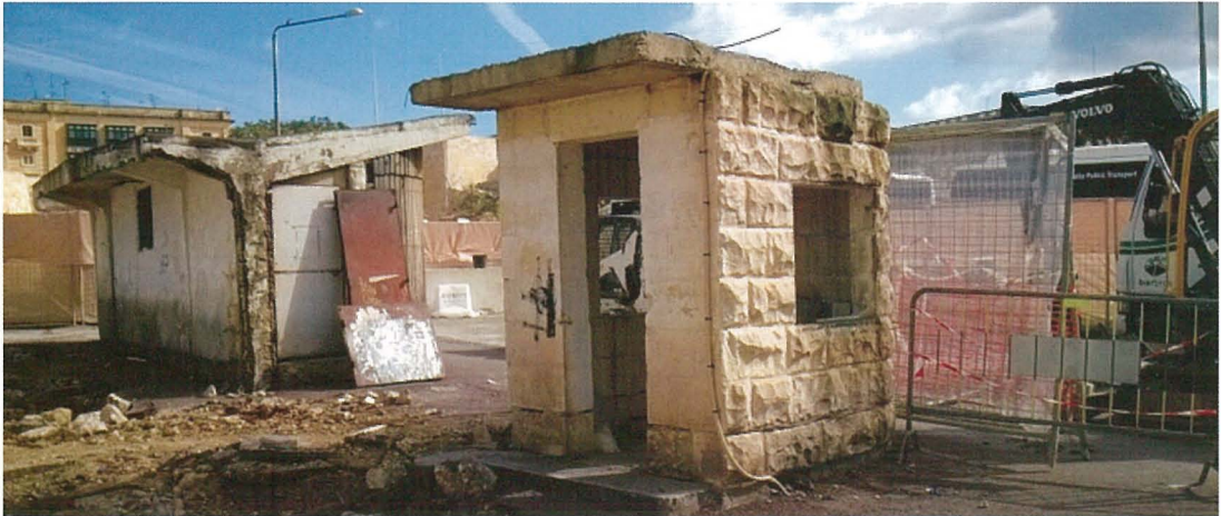
Demolition works of old and derelict kiosks. GHRC
