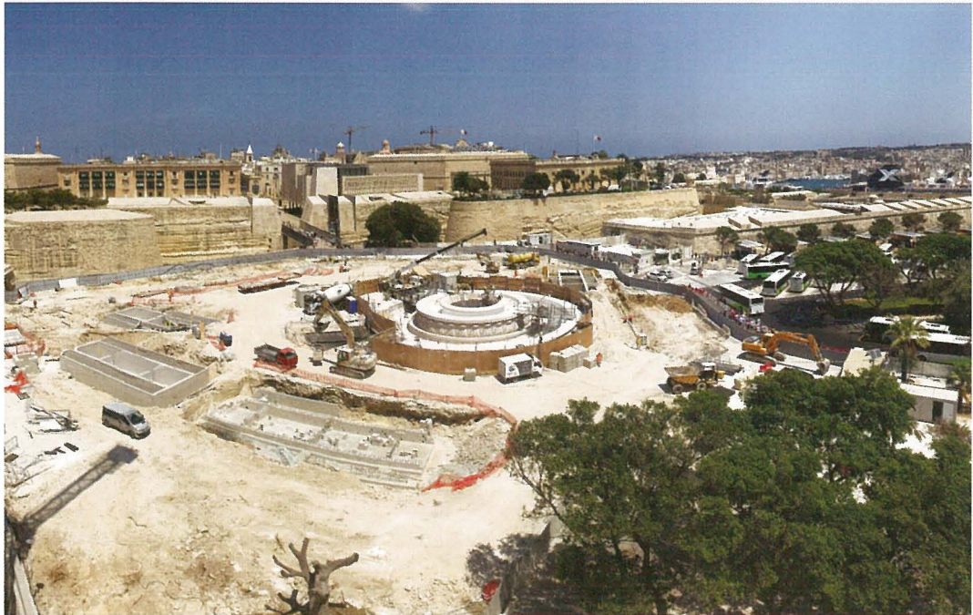
Groundworks in progress at Triton Square. GHRC
