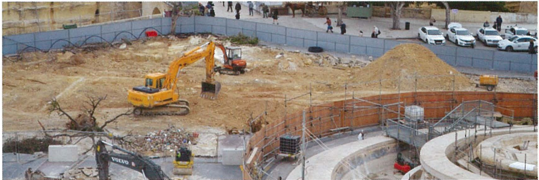
Surface excavations and other groundworks. GHRC.
