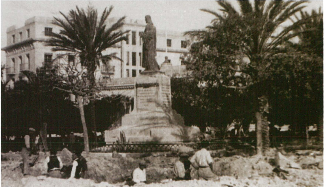
Workers repairing WWII bomb damage adjacent to Christ the King statue, c1948. DOI.
