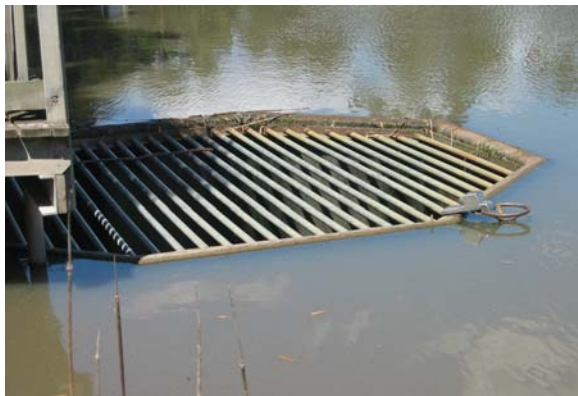
In contrast, the vertical drop structure with grille (left) would be impassable to a platypus – forcing dispersing animals to leave the associated lake and move across land to travel downstream.
