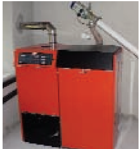
Wood pellet central heating boiler
