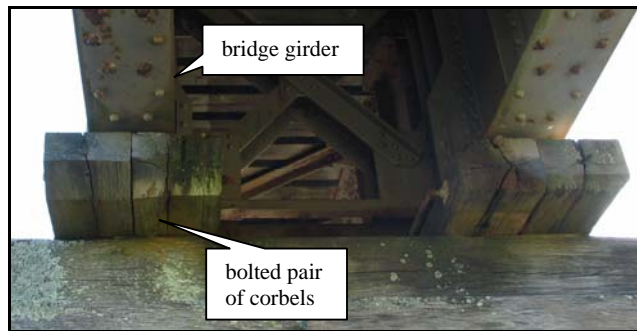
Figure 7 Close-up of corbel and girder arrangement
