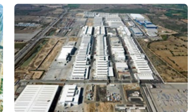
33 SUZUKI MOTOR GUJARAT PRIVATE LIMITED (Gujarat Plant)
