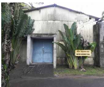
The then PED building which currently houses the motor assembly hall and burning rate lab
