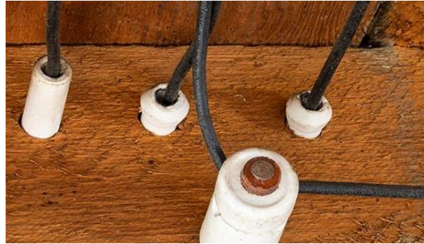
Wire and Tube Wiring system
