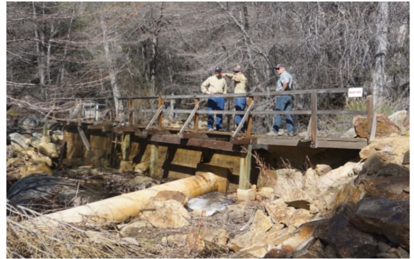
Salmon Creek Diversion
