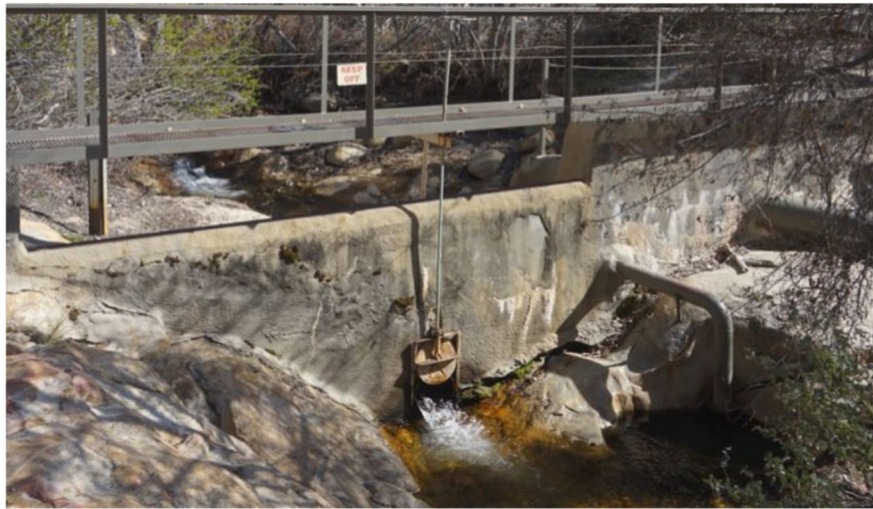
Corral Creek Diversion
