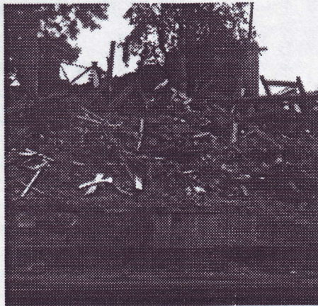
Above: late 19thc building collapses on itself through lack of interest. The only other European city where this happens regularly is Lisbon
