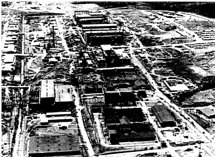
Figure 3. Construction of the electromagnetic complex called Y-12 was underway by 1943 at the top-secret Clinton Engineer Works in eastern Tennessee. In time, more than 1,100 calutrons were operating there, a process that required persistent troubleshooting and design changes to optimize an experimental technology that had never been scaled to industrial use. (Photograph courtesy of Y-12 National Security Complex.)
