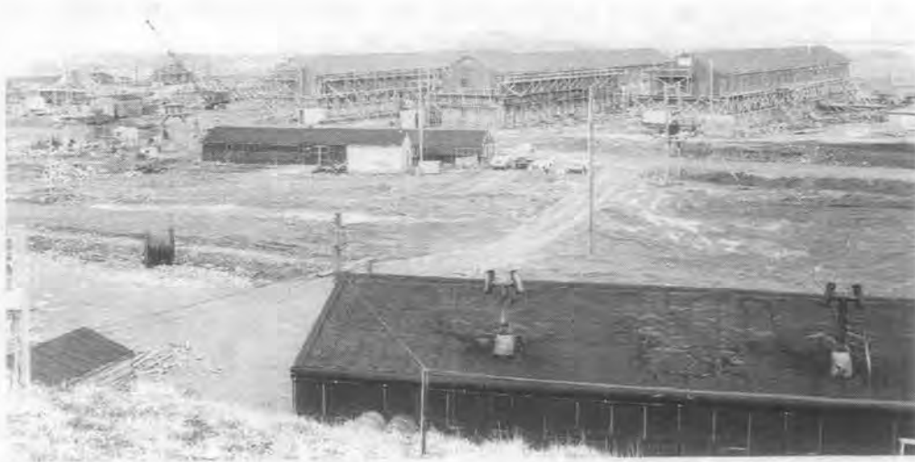
Permanent barracks being built at Davis Air Force Base, Adak.
