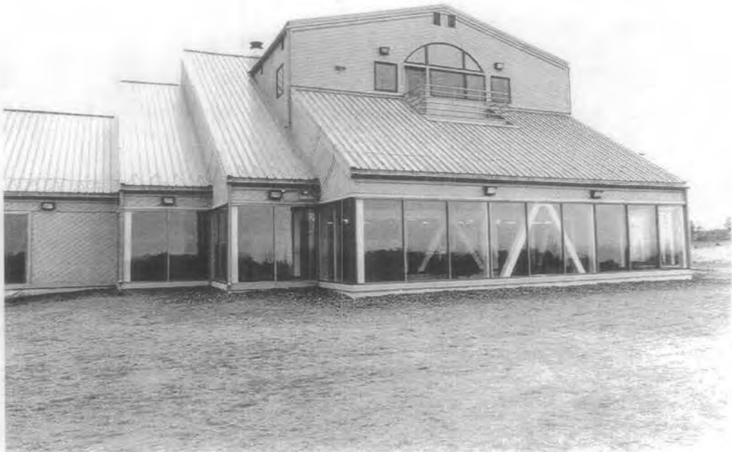
A Site Point launch structure was effectively made into a lodge.
