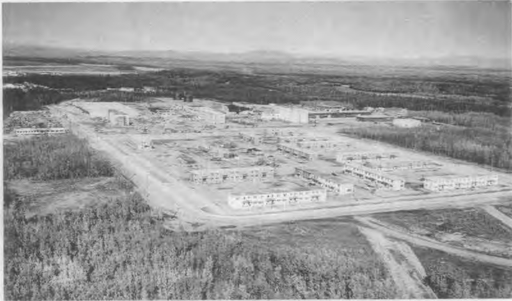
Fort Greely under construction in the early 1950s
