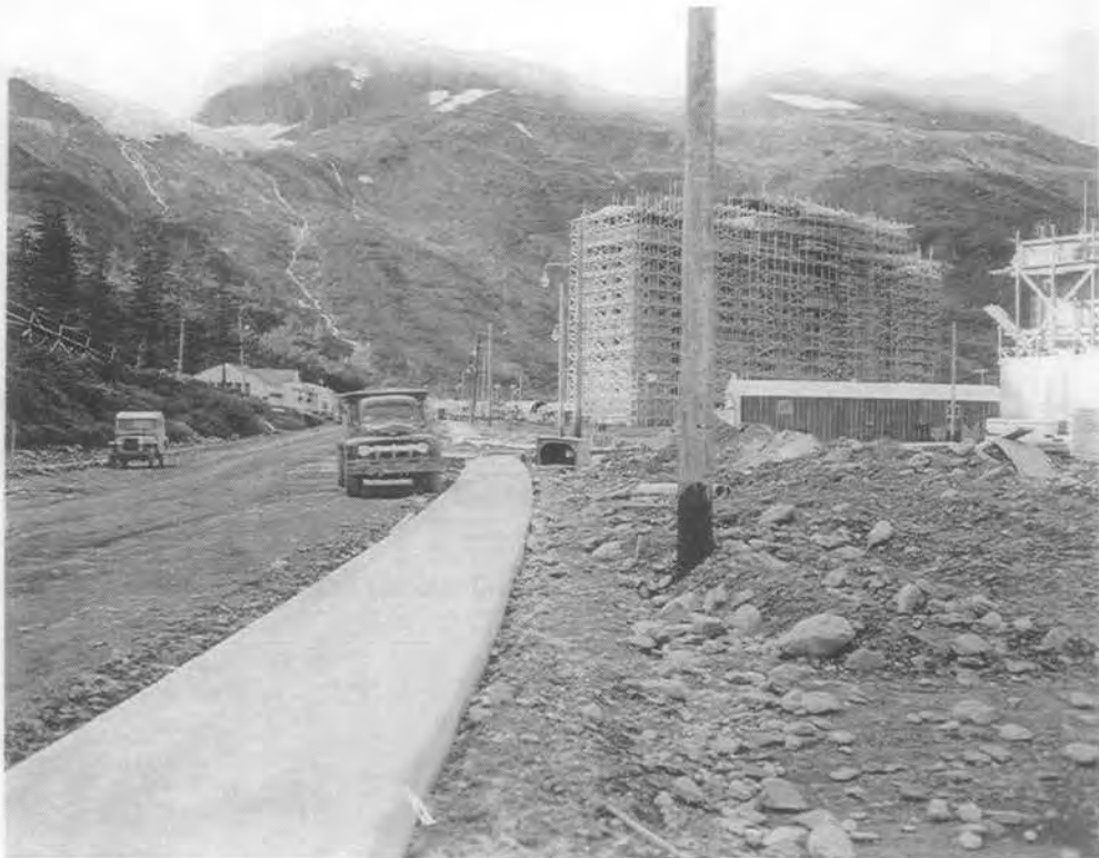
Hodge Building under construction at Whittier.
