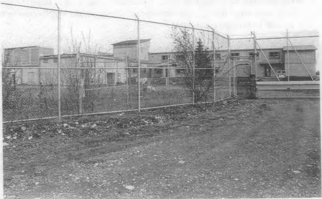
The Site Bay correctional center was operated only a short time and then closed. Despite the high security fence, the building has been heavily vandalized.
