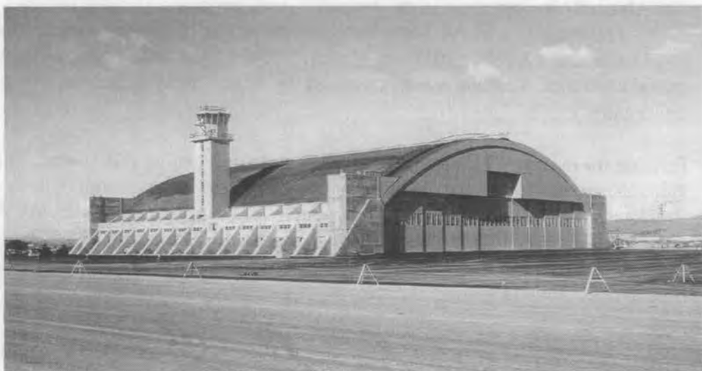
Largest hangar in Alaska is erected at Eielson AFB.
