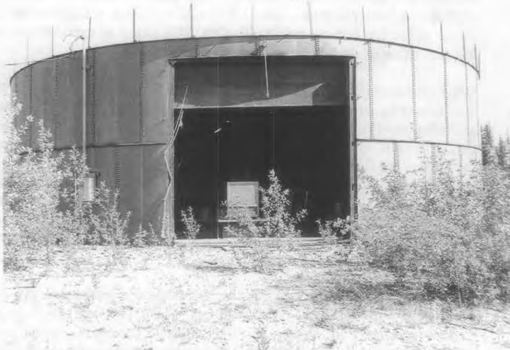
An above-ground fuel tank at Gulkana was given a door to convert it into a garage.
