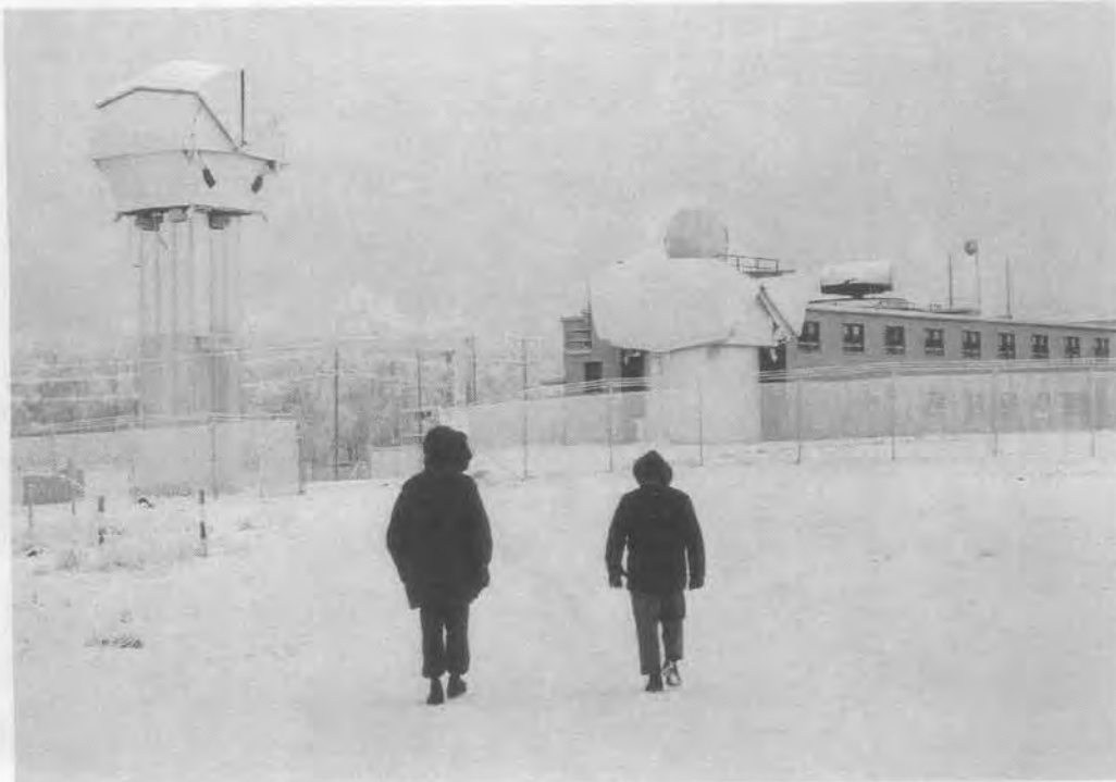
Winter day, 1962, at control building at a Nike installation near Fairbanks.
