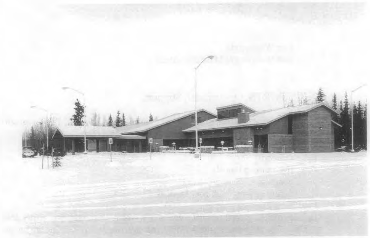
New club at Fort Wainwright, 1994. (photograph by Brian Allen)
