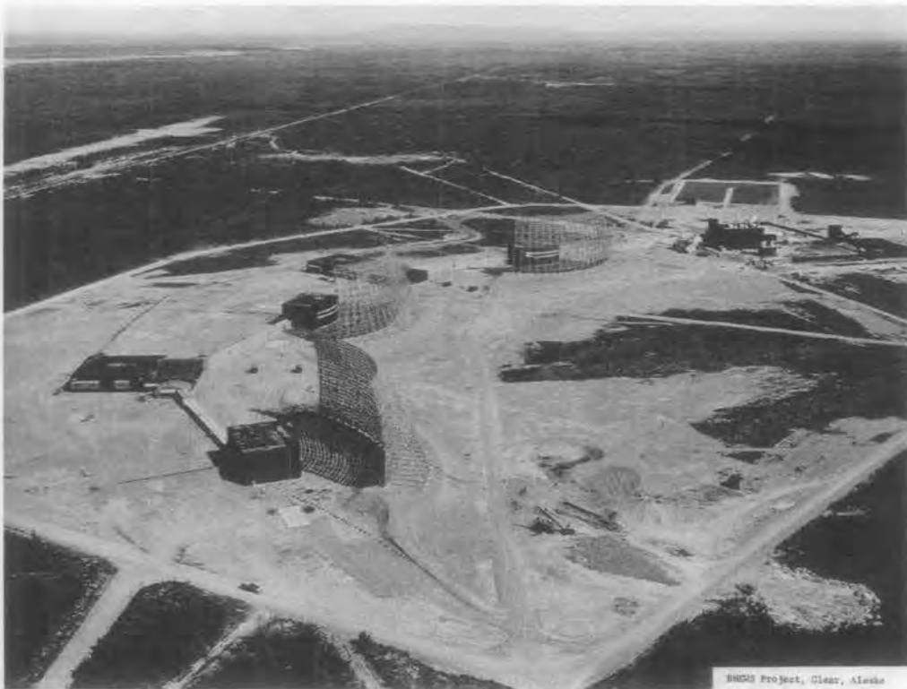
The Ballistic Missile Early Warning Station at Clear nears completion in 1959.
