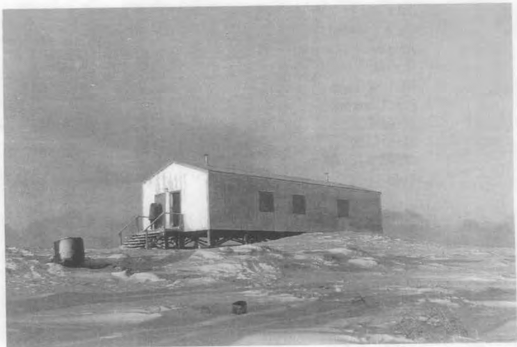
Alaska Army National Guard armory at a remote village.
