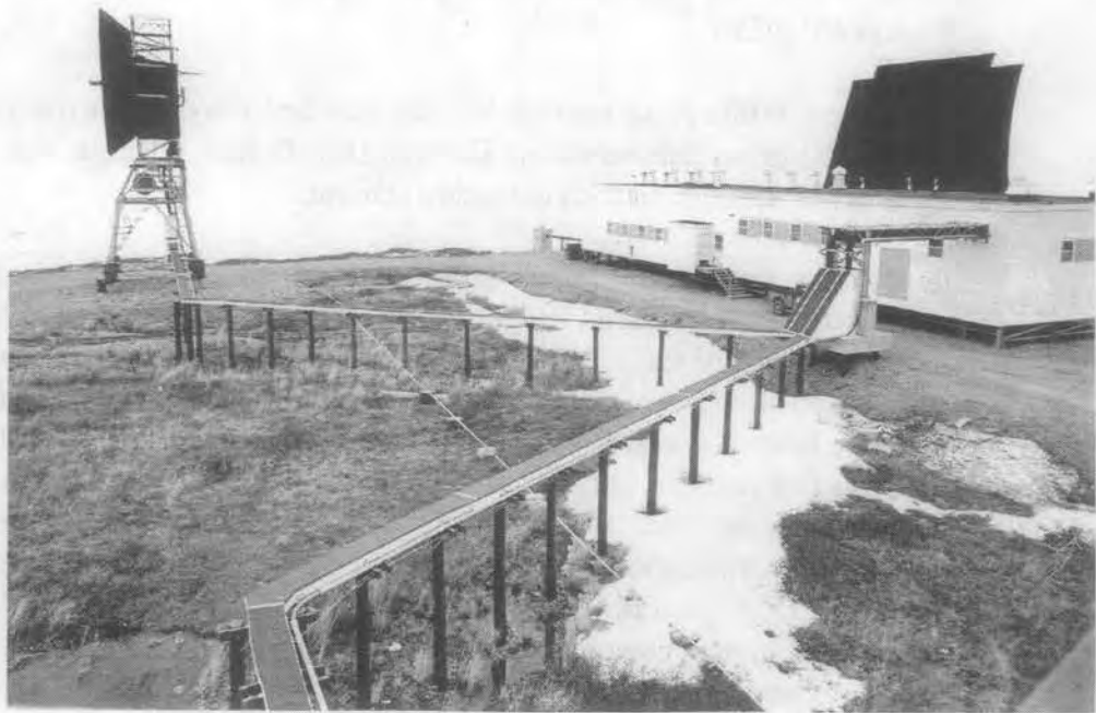
Kotzebue White Alice equipment building.
