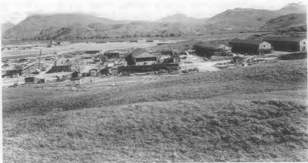
Permanent barracks construction at Sweeper Cove, Adak.
