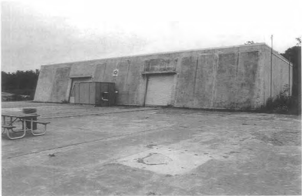
Nike Hercules launch structure serves as a storage shed at the former Site Point, Anchorage.
