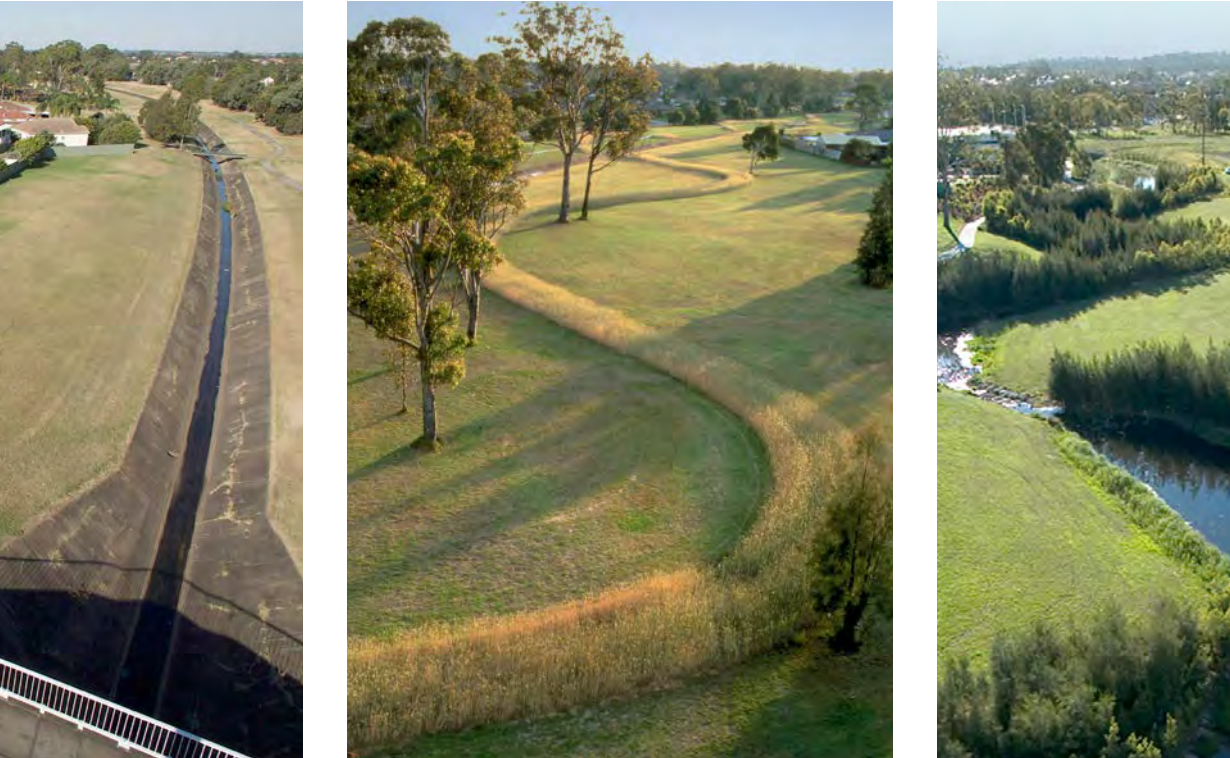
The restoration of Clear Paddock Creek (Schaffer Barnsley Landscape Architects with Turpin Crawford Studio).
