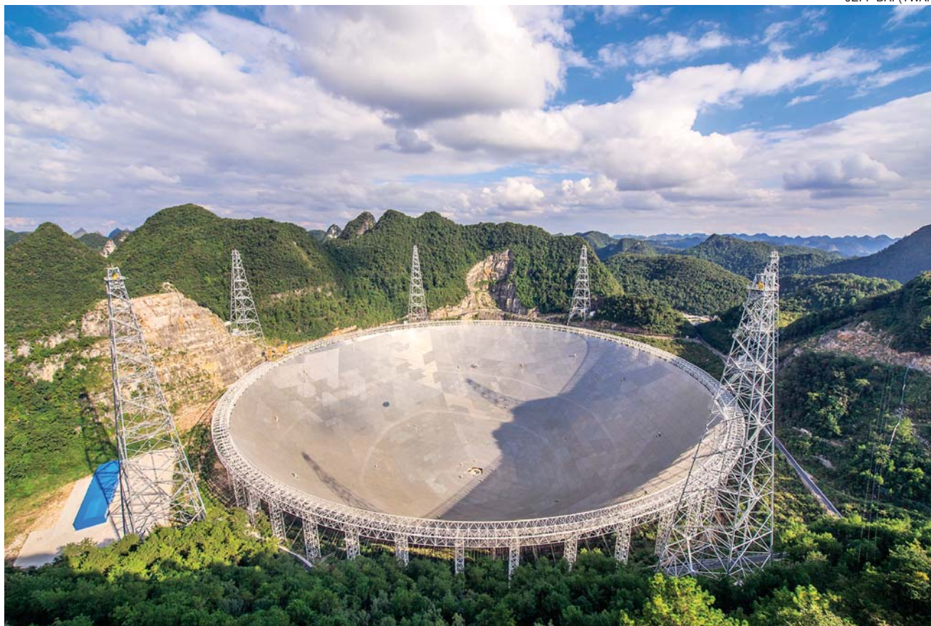
FIGURE 2. THE WORLD'S LARGEST filled-in, single-dish radio telescope, the Five-Hundred-Meter Aperture Spherical Radio Telescope in Guizhou Province, China, entered its commissioning phase last September. Despite the telescope's fixed gaze on a relatively small patch of the sky, the National Astronomical Observatory of China plans to use it to search for potential signals from intelligent life beyond Earth.
