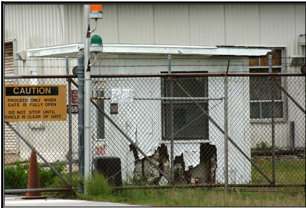
Figure 77. View to the southeast of Facility 18803.
