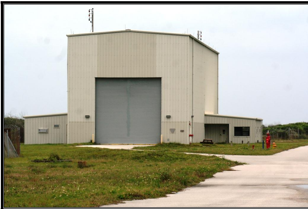
Figure 63. View to the northeast at Facility 18705.
