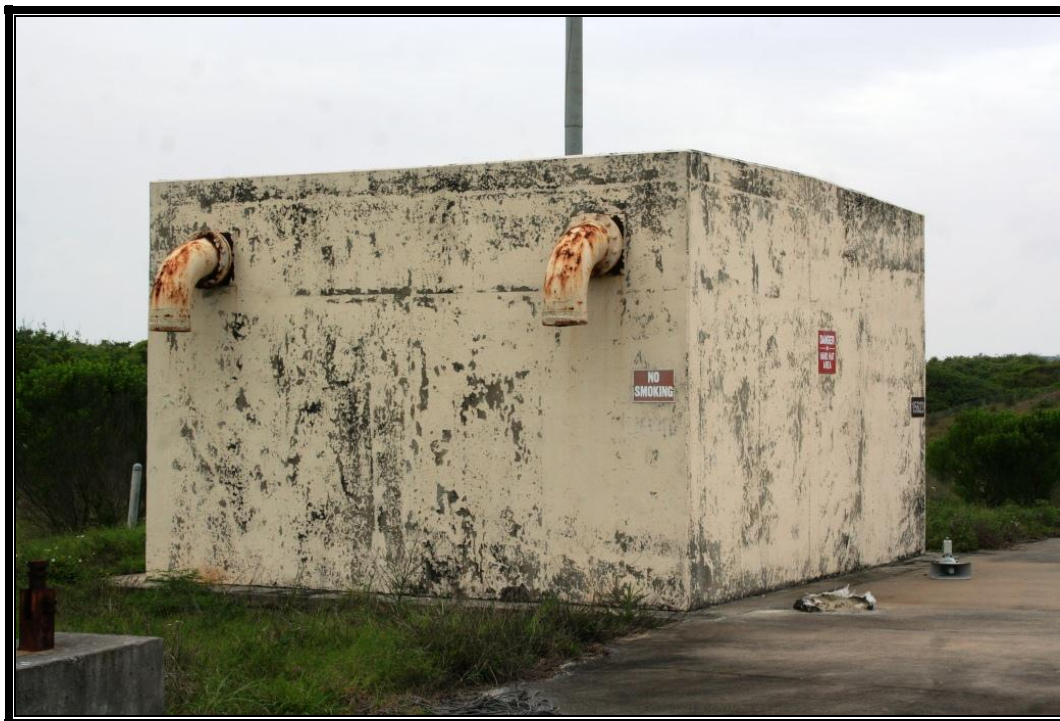
Figure 61. View to the west of Facility 15641-Equipment Building.
