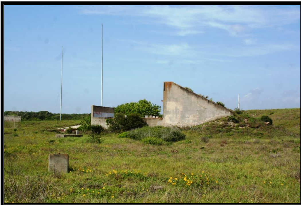
Figure A-4. View to the west of Facility 15500AD.
