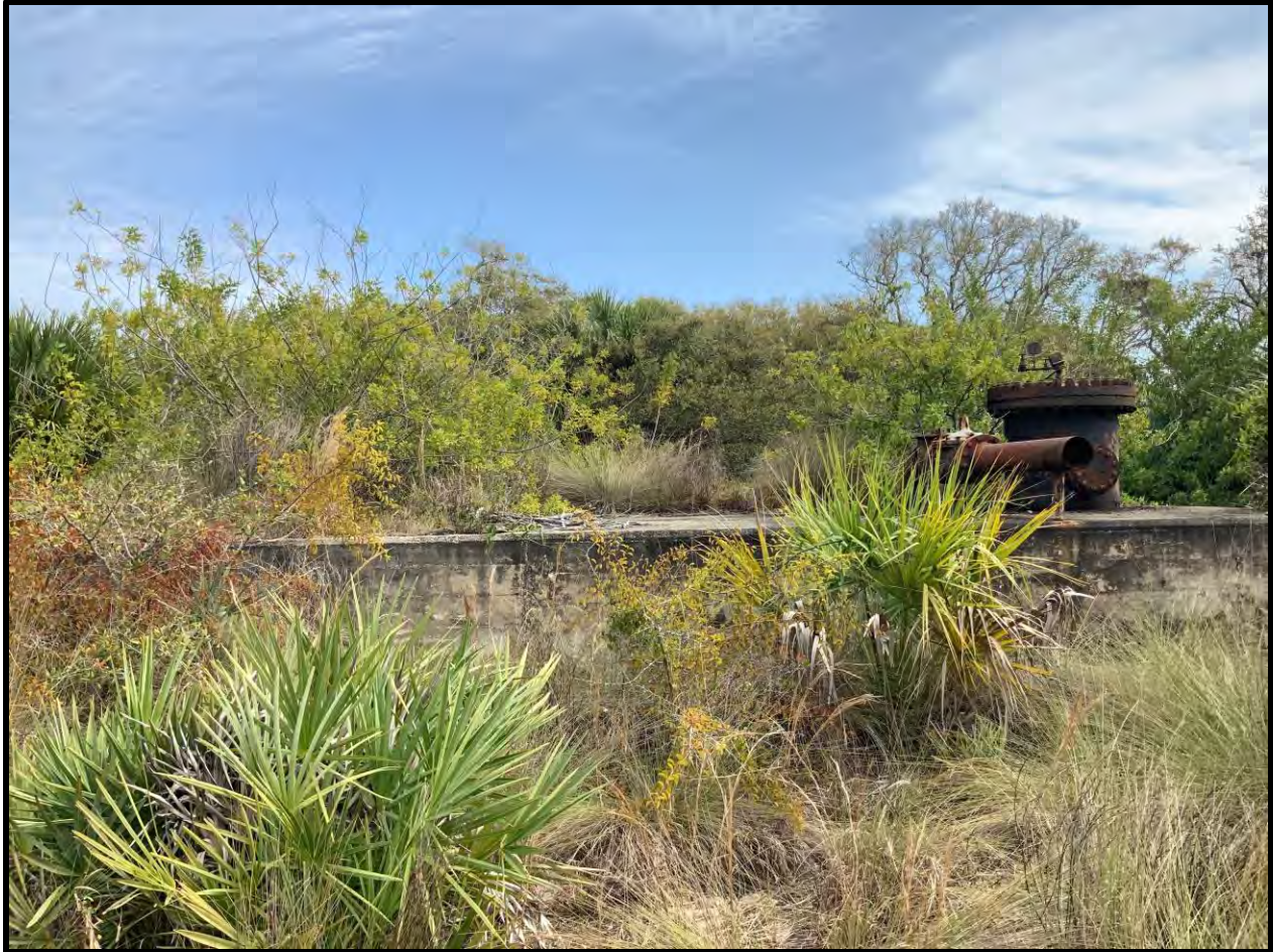
Figure 11. Similar structure to the one found in LMU 15. Preliminarily identified as a Thrust Block and Valve Pit - view facing N.
