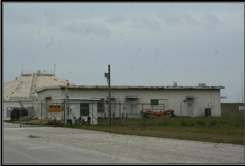
Figure 81. View to the southeast of Facility 18806.
