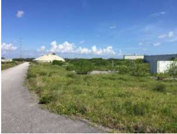
Photograph 5-1 South Side of SLC-20
