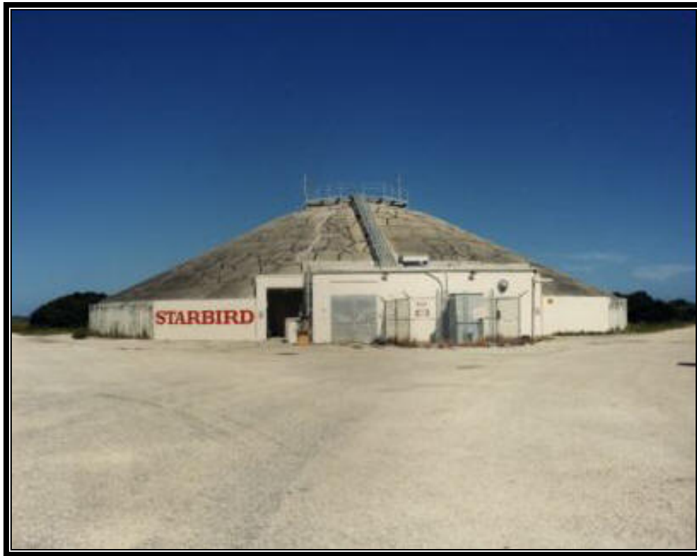
Figure 68. View to the west of the LC-20 Blockhouse during the Starbird program (Bionetics Corp. 1990).
