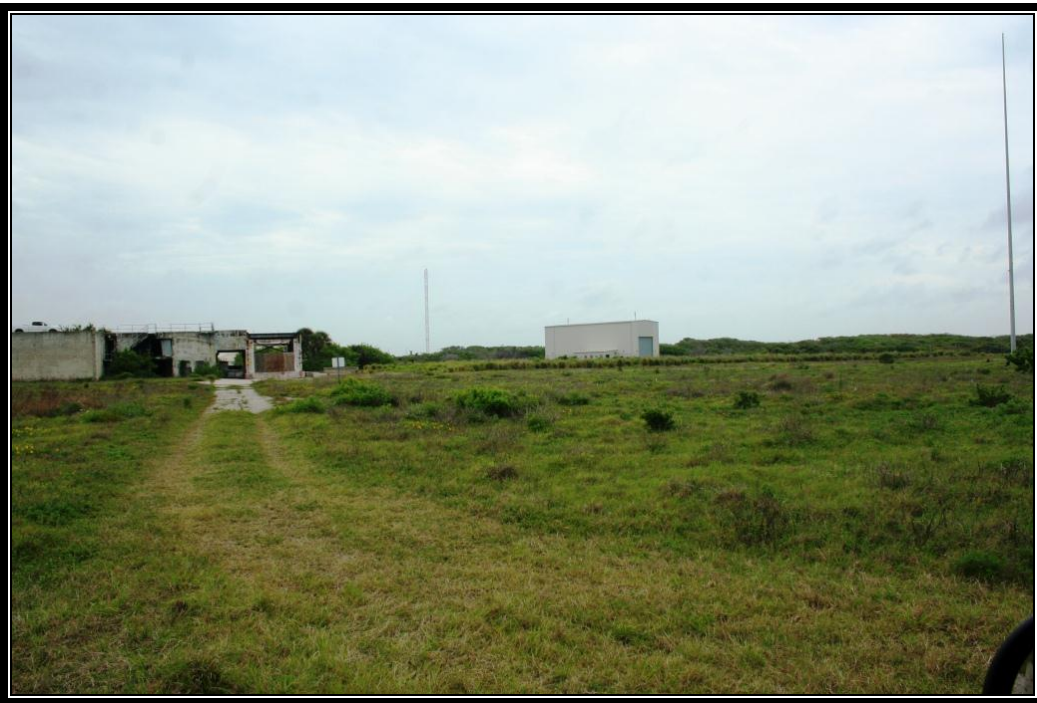
Figure A-2. View of the Launch Stand and Ramp and Facility and Warehouse.
