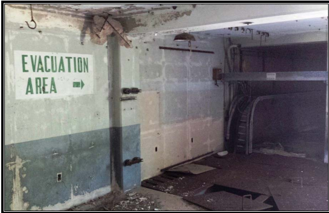
Figure 45. Interior photograph of Facility 15500B showing current conditions.
