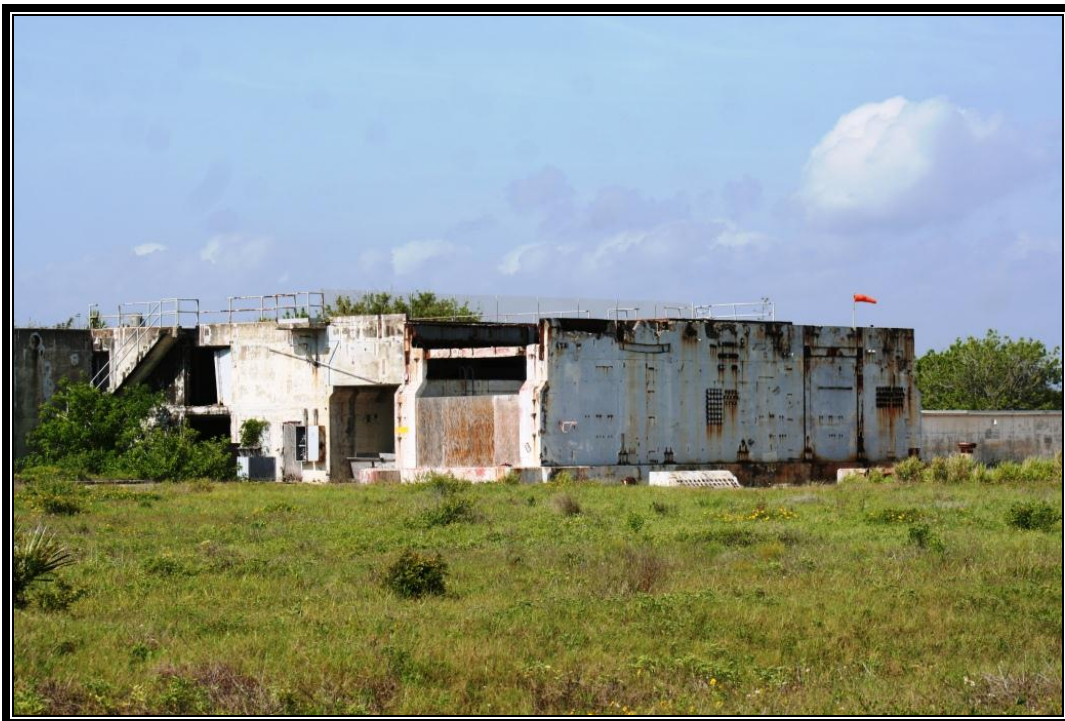
Figure 44. View to the southwest of the main section of Facility 15500B.
