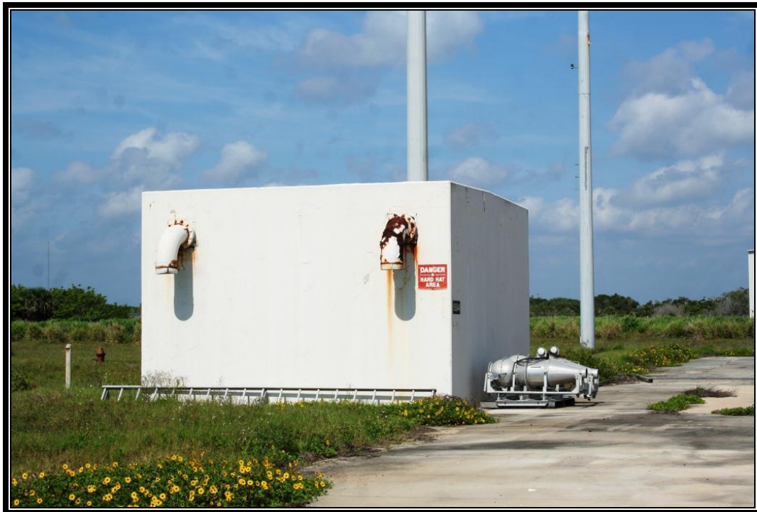
Figure 53. View to the west of Facility 15541-Equipment Building.
