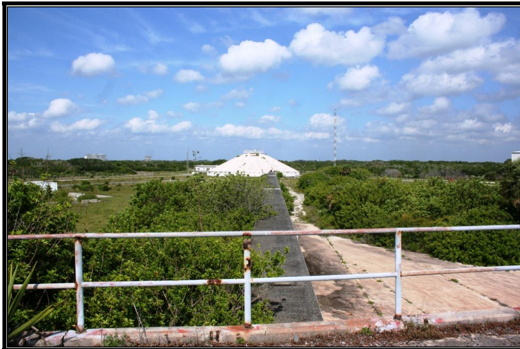
Figure 28. Photograph from the top of the Launch Stand and Ramp of Facility 15500-Control Cableway (8BR3151), looking west.
