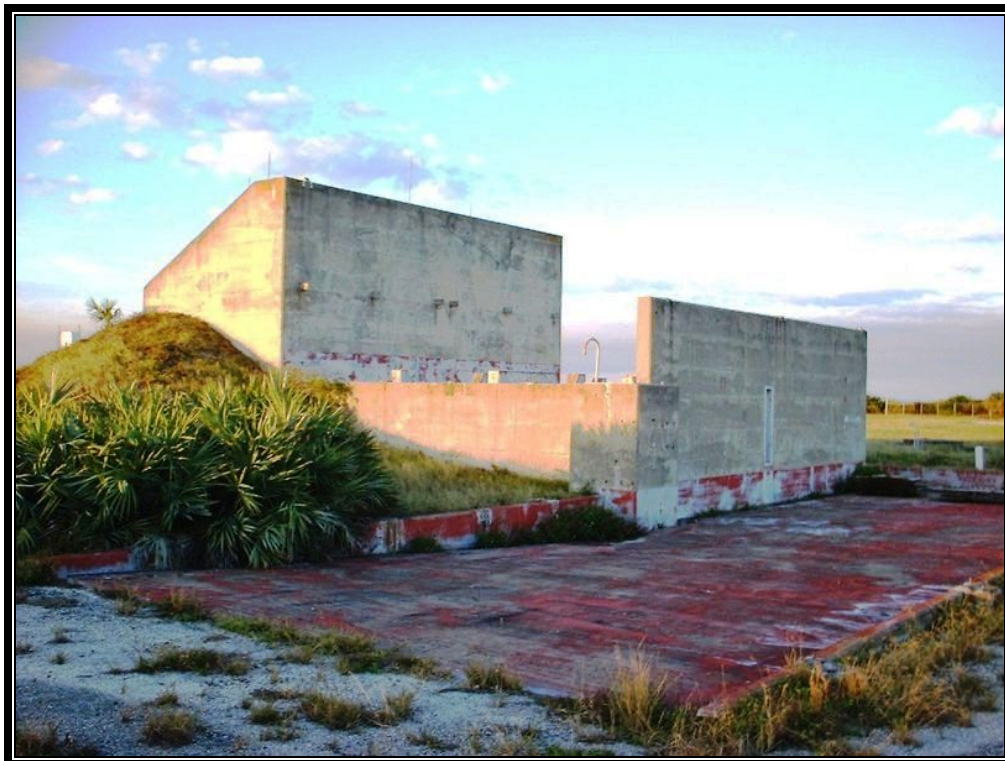
Figure 31. View to the northwest at Facility 15500AD-Liquid Hydrogen Holding Area (8BR3152).
