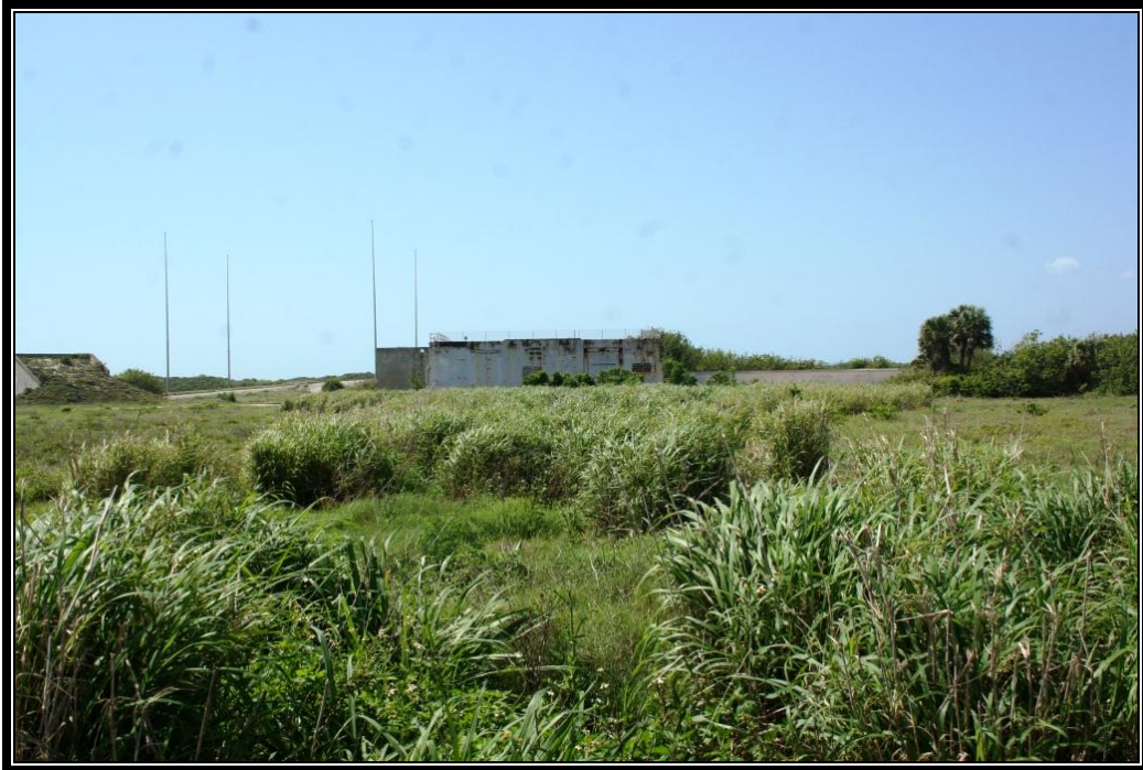
Figure A-1. View to the south of the former flume and basin.
