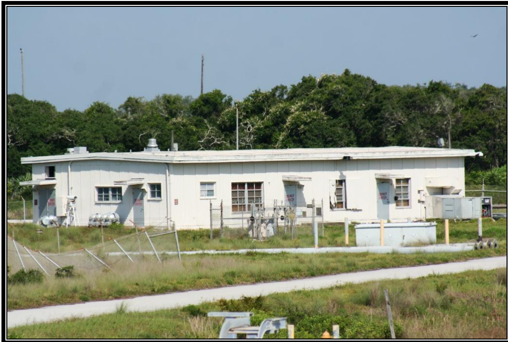
Figure 82. View to the northwest of Facility 18806.
