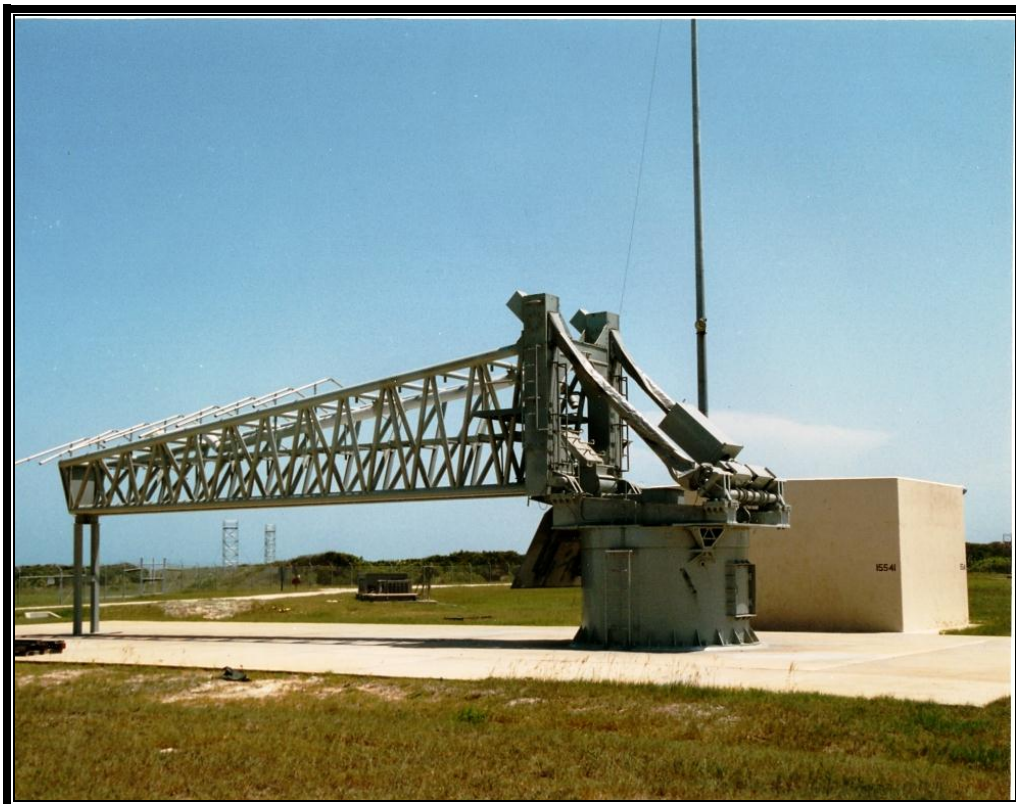
Figure 49. Photograph from 1993 showing Facility 15540-Launch Pad A-BMDO (Bionetics Corp. 1993a).
