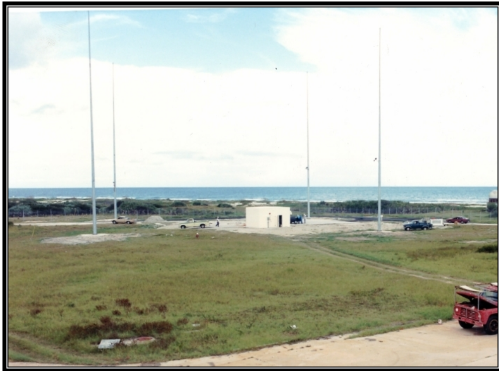
Figure 48. Photograph from 1989 showing Facility 15540-Launch Pad A-BMDO under construction (Bionetics Corp. 1989a).
