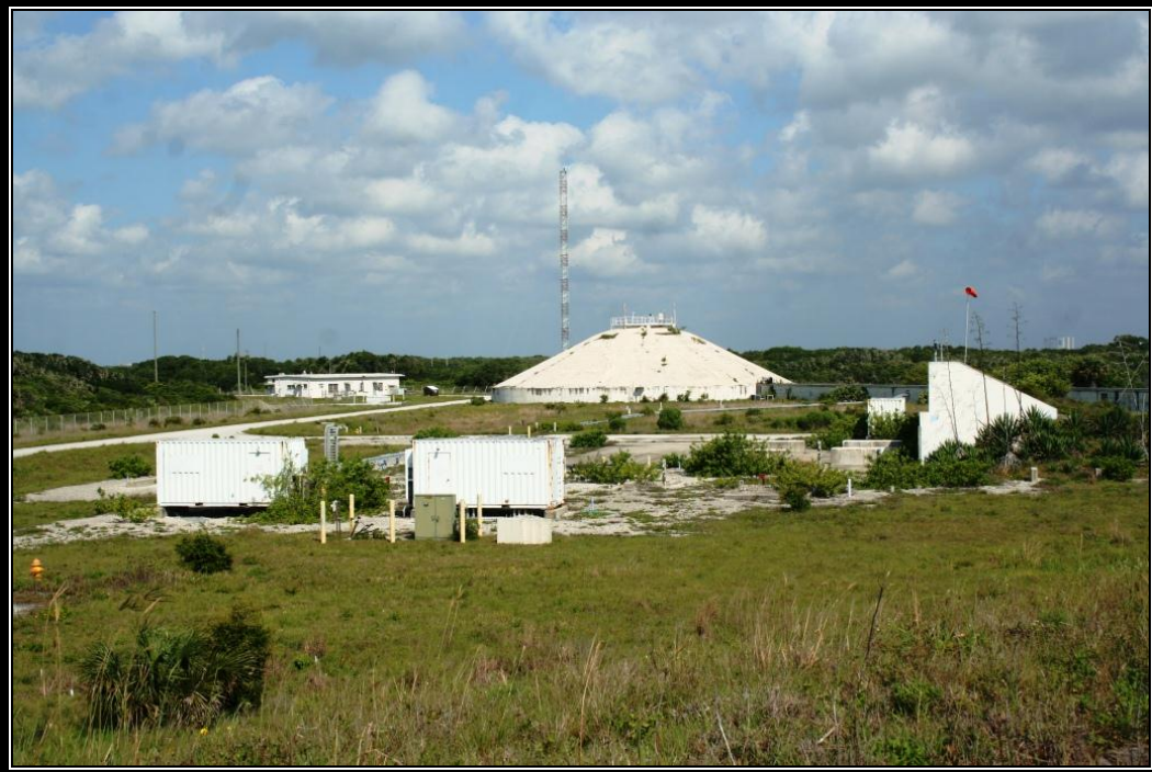
Figure 37. View to the west of the Facility 15531 area.
