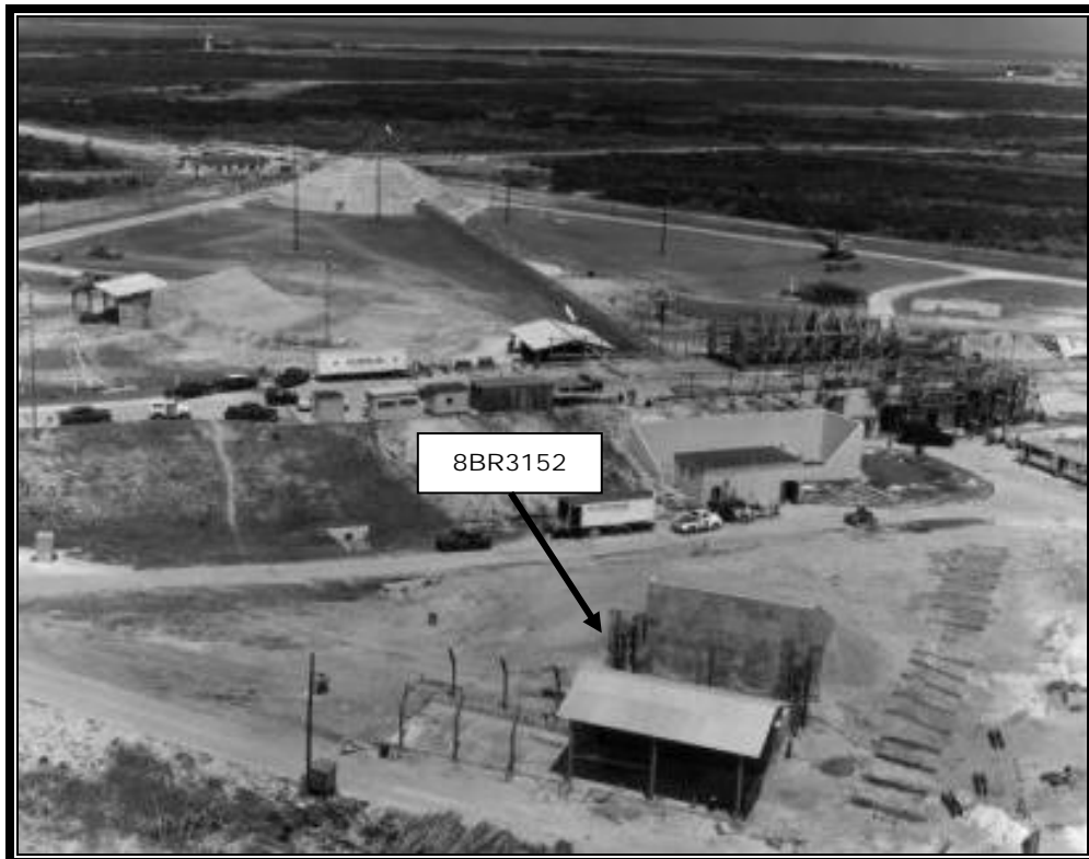
Figure 30. Photograph from 1963 showing LC-20 undergoing renovations with Facility 15500AD-Liquid Hydrogen Holding Area (8BR3152) in the foreground (Photograph courtesy of the AFS&MM).
