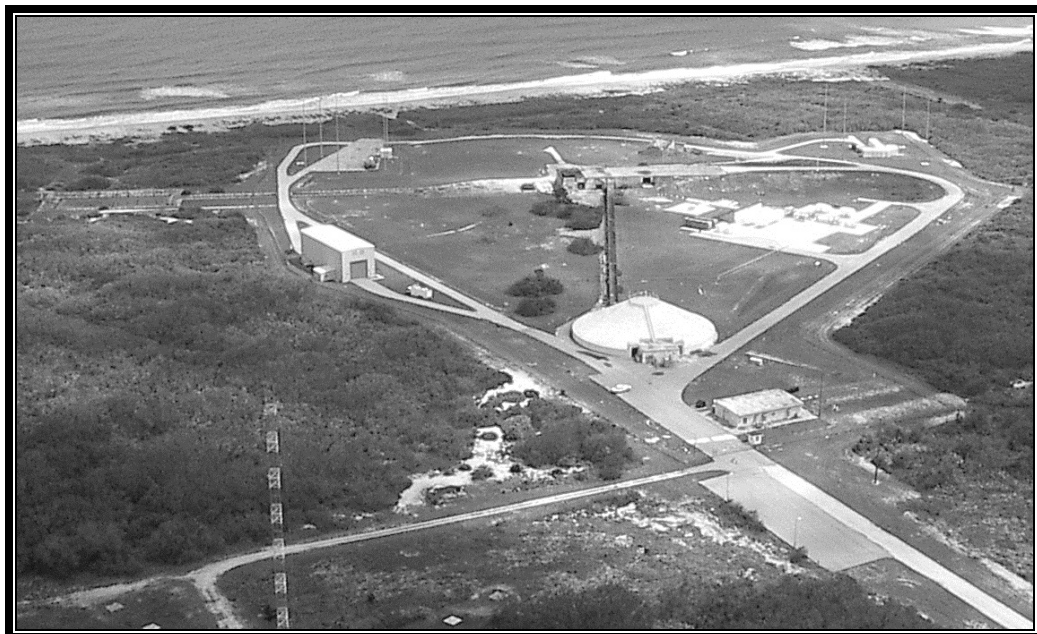
Figure 36. View to the east of LC-20 from 2005 (SGS 2005).
