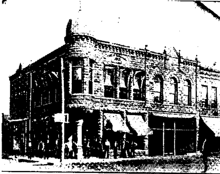
Figure 17. The First National Bank Building as it appeared in the early 1900s. Photo courtesy The Planter's Trust Company, Glimpses Through Holdenville and Vicinity , 1904, page 22.
