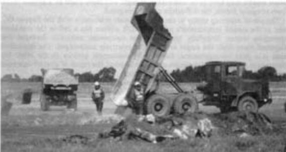
Photo 4. Placing the fill
