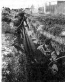
**Photo 5** The Stanley water main from Moody Brook treatment plant to Dairy Paddock reservoir. Dewatering in progress
