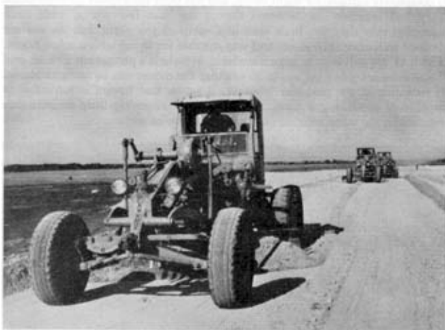
Photo 7. Three BK 12 graders produced an excellent surface.
