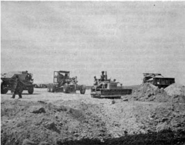
Photo 6. Spreading, and forming the runway.
