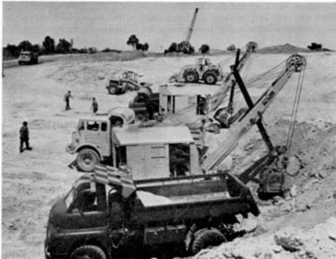
Photo 2. Early days in the quarry. The tippers are (from front) an ex-RAF 3 ton Bedford, an Army 10 ton AEC, and an ex-RAF 7 ton Bedford.
