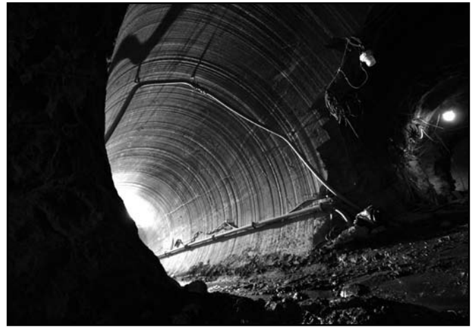
An image by Hiroyuki Suzuki of an East Side Access tunnel.
