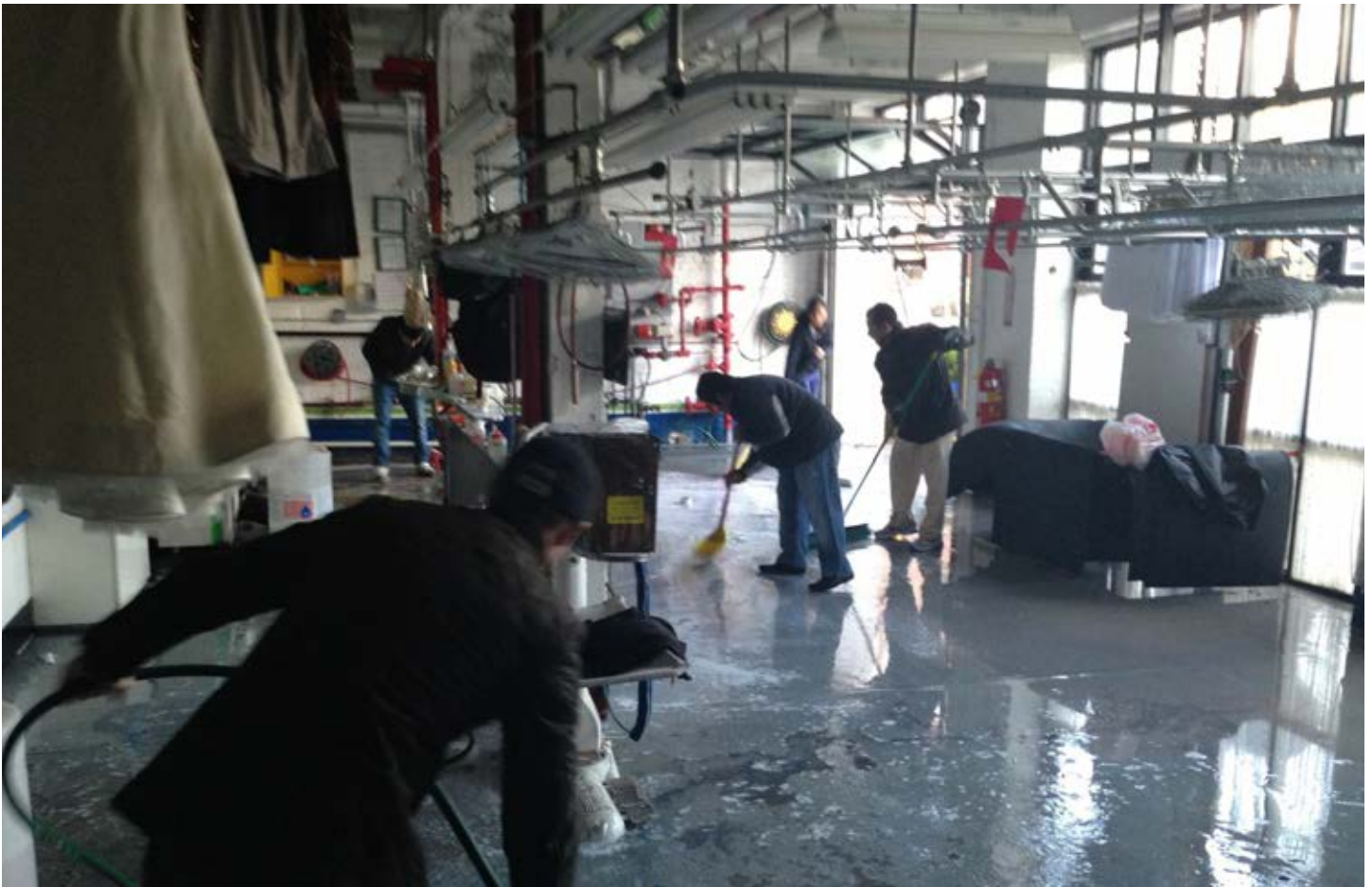
Repairing damage at a flooded dry cleaning facility following Hurricane Sandy.
