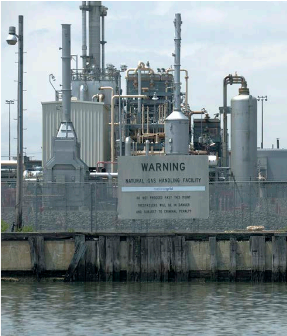
Petrochemical facility along Newtown Creek in North Brooklyn.
