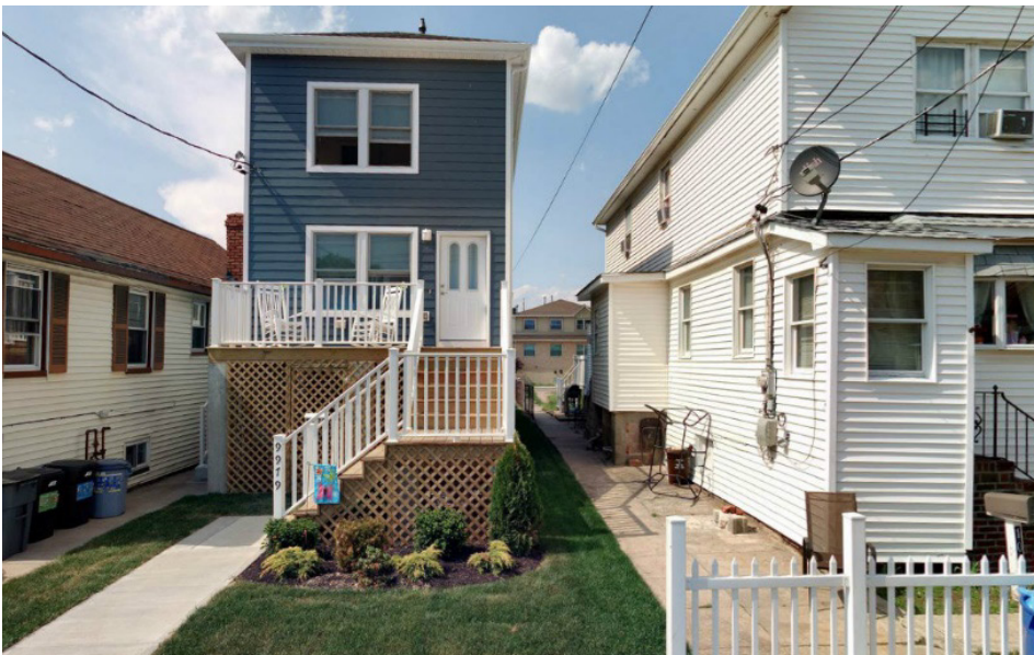
Building rebuilt under 2013 Flood Text Location: Queens
