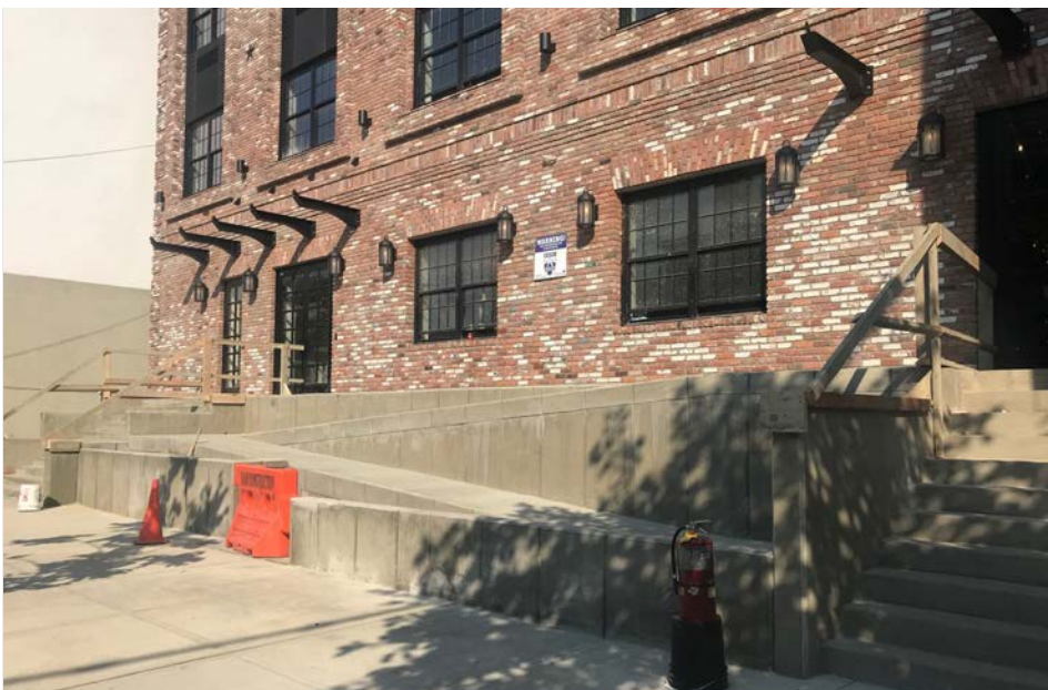
Elevated access with extensive ramps in residential neighborhood Location: Brooklyn
