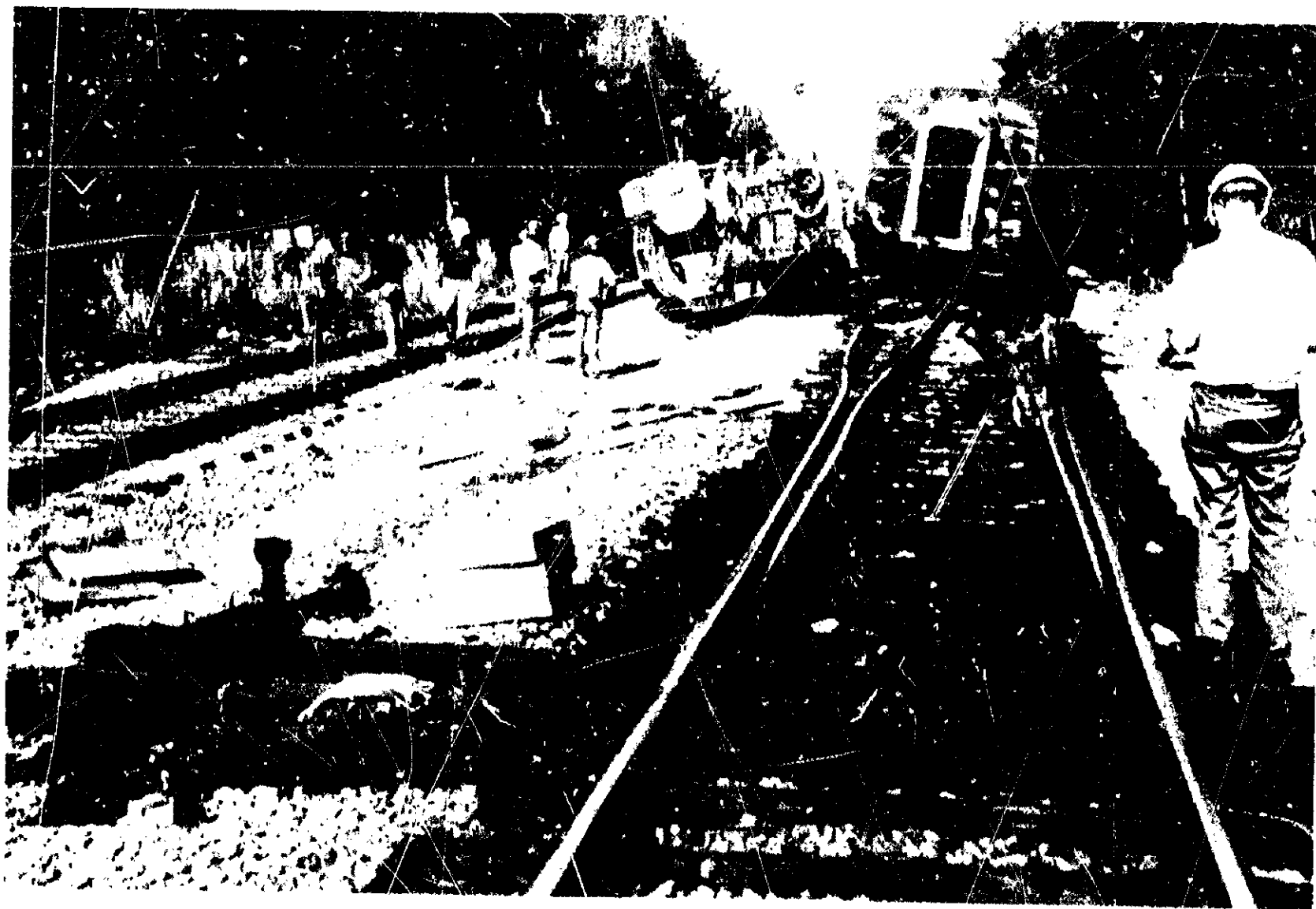
Figure 5.—Westbound turnout at Juniper.
