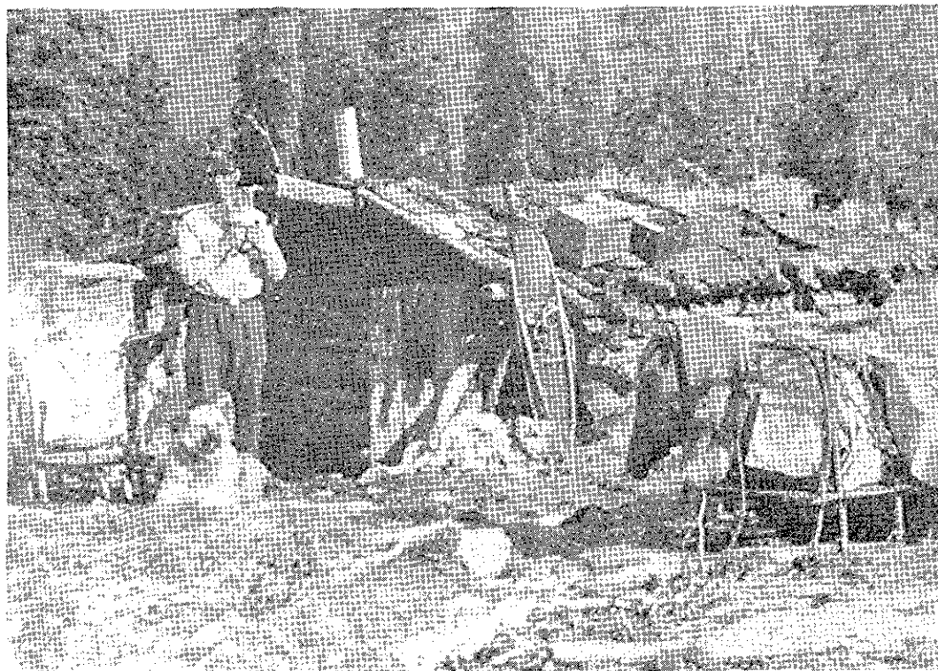
Old Market Hunters' Shelter used by early park rangers for night shelter. 1926.
