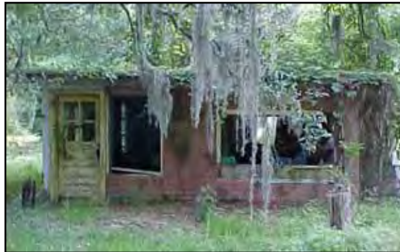
This 100 year-old structure was once Boney Brown's Store and family residence on Squire Pope Road, Hilton Head Island, SC. Although the Brown-Grant family had hoped to save the building, it was recently demolished.
