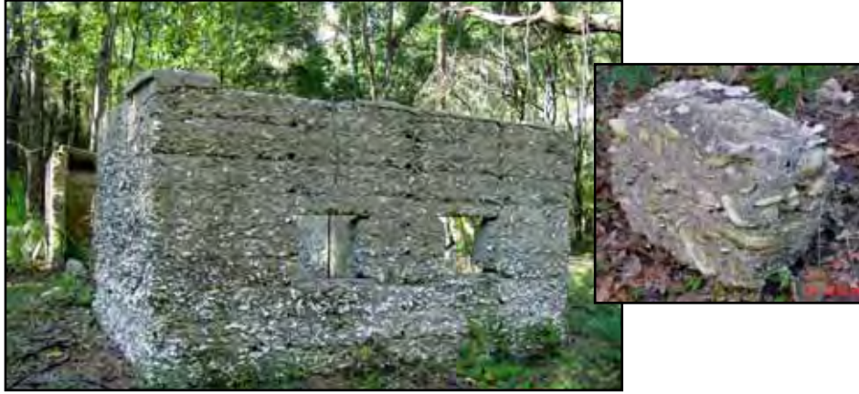
Tabby ruins are all that remain of the old sugar works and rum refinery at the Thicket, Carnochan Creek, near Darien, McIntosh County, GA.
