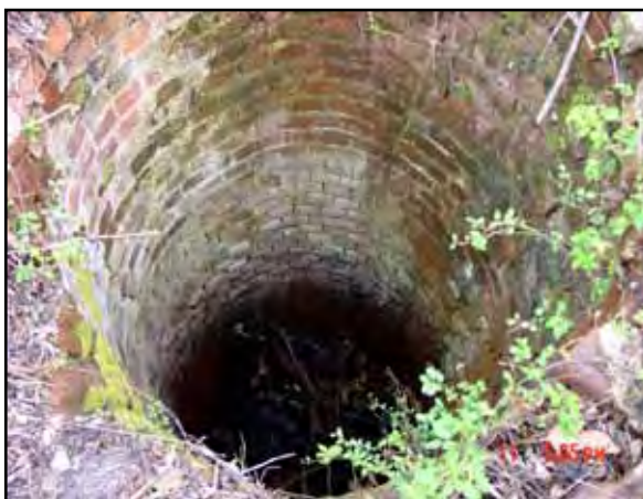
One of two abandoned wells in the Phillips Community. Well was constructed with bricks handmade on Parker Island, which is now River Town Country Club.
