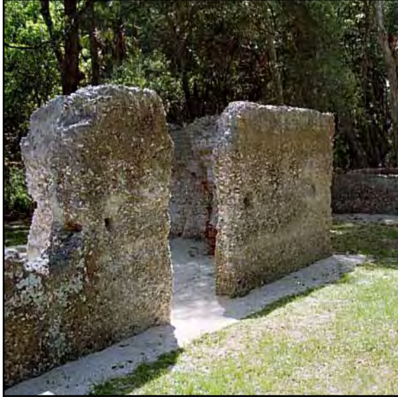
Ruins of tabby slave cabin, Kingsley Plantation, Timucuan Ecological and Historic Preserve, near Jacksonville, FL.
