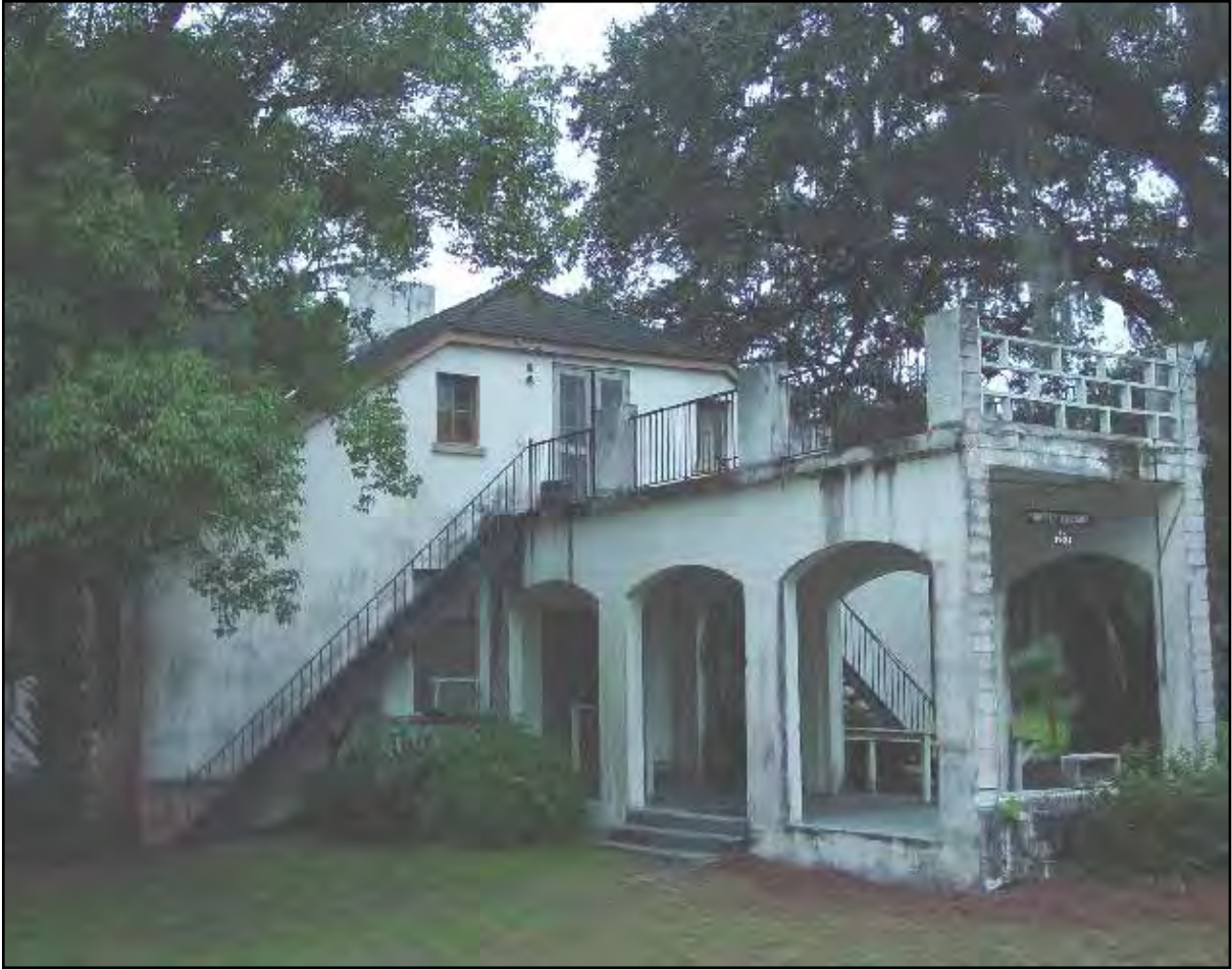
Butler Building, Penn Center, site of possible museum/curatorial/learning center facility.
