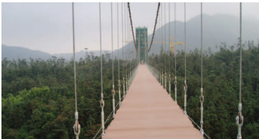
WPC is progressing: suspension bridge with WPC boards. Picture: China Wood-Plastic Composites Union (CWPCU)
