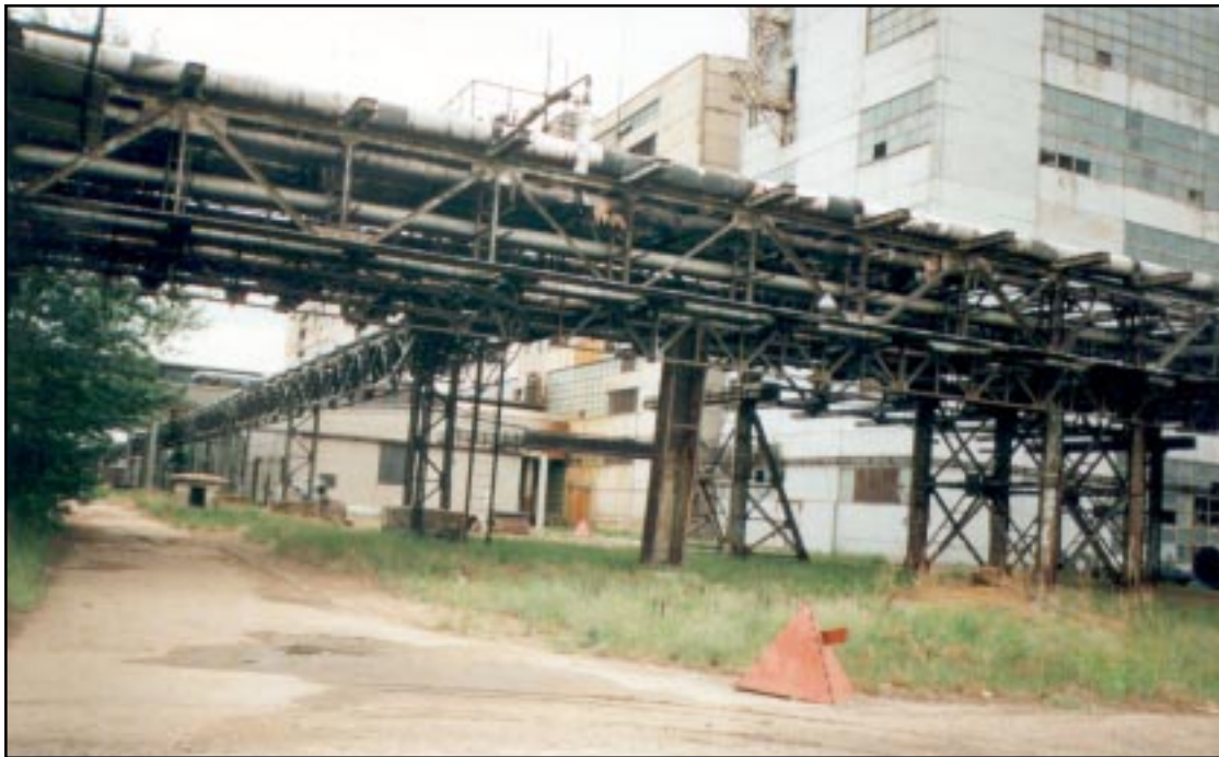
Figure 2: Pavlodar Chemical Plant, Site Number Two, intermediate precursor production building
