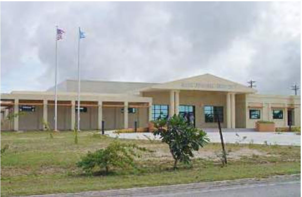
The Rota Judicial Center has courtrooms for the Supreme Court and Superior Court and also provides offices for the Attorney General and Public Defender.
