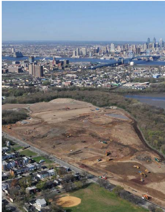
The former Harrison Avenue Landfill during remediation.
