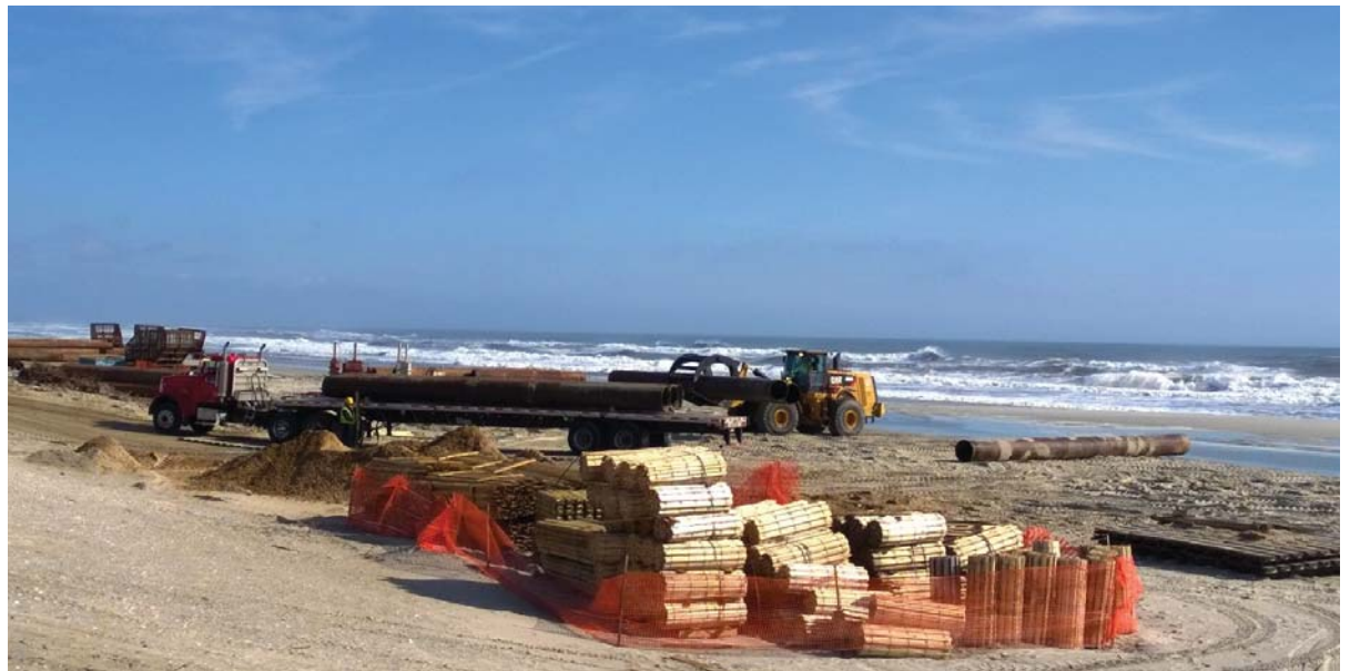
Beach construction along the Jersey Shore.
