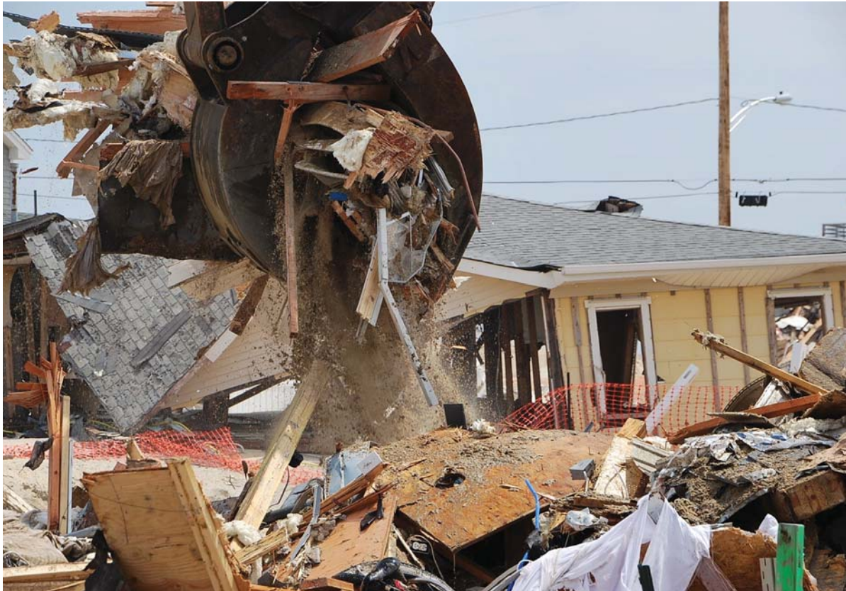
Home demolition in Ortley Beach.
