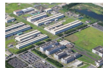
Research & Engineering Center (Futtsu)
