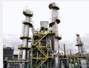
AIR WATER CARBONIC INC.
