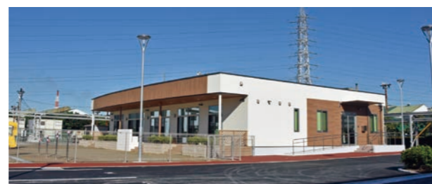
In-house childcare center (Nagoya Works)
