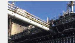
Muroran Works No. 5 coke oven (CO) refurbishment
