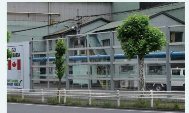
Transparent plates installed at the border in the East Nippon Works Kamaishi Area
