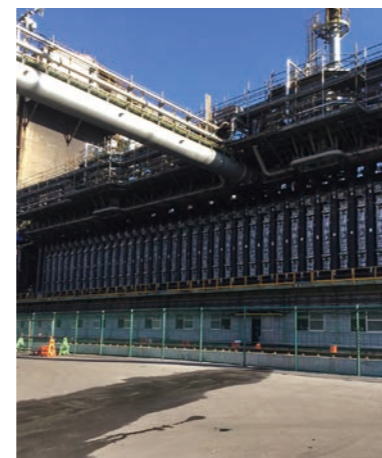
Muroran Works No. 5 coke oven (CO) refurbishment
