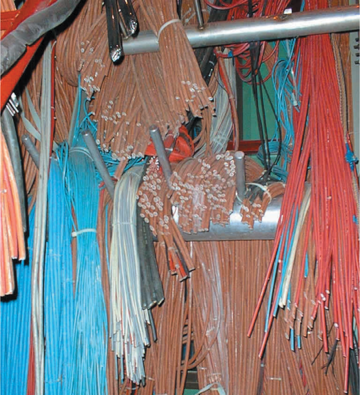
Dismantling of the DELPHI detector.
