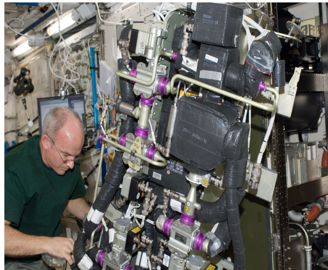
Crewmember performing maintenance on ISS CDRA
