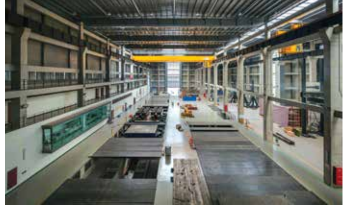
Tongji's MFST Lab features two 70-ton shake tables and two 30-ton shake tables that can be arranged in multiple configurations anywhere within two adjacent trenches.
