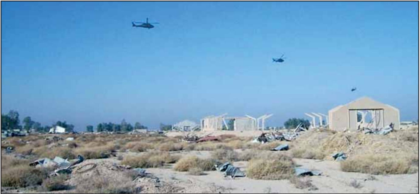
“One of the properties was a large compound that had been used for storing rockets. It was extensively bombed during the invasion and consisted of two large derelict hangar-type buildings, dirt roads, and smaller bermed areas where rockets were stored. With the exception of the two destroyed hangars (for more of an urban setting), it was an excellent area for tank driver training and a dry fire TCPC range.”
