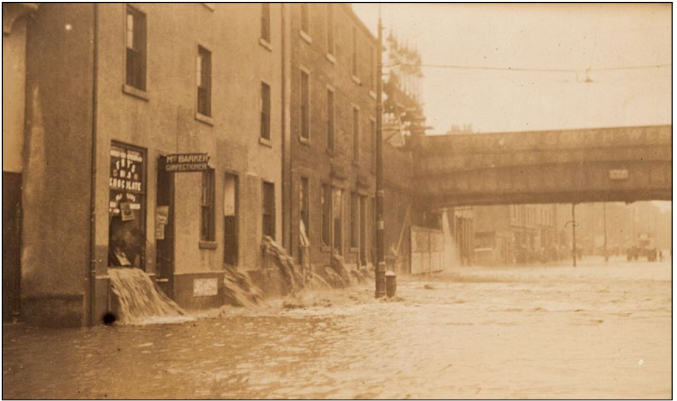
Tenements between the railway bridge over Brougham Street and Robertson Street after the bulk of the flooding had subsided, although water still pours from the shops and houses at street level.
