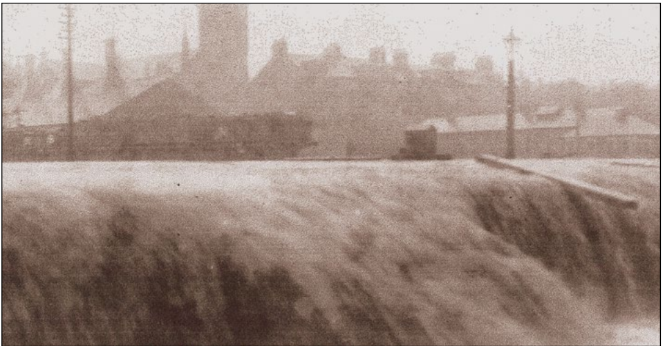
The scene at the railway sidings where the water which had poured through the tunnel from Inverkip Road was still cascading down towards the tenement in Brougham Street. In the left background, behind the coal wagons, was the Glasgow & South Western Railway engine shed at Greenock (Princes Pier). This photograph was believed to have been taken when the flood was at its height from a position in the Picture Palace Picture House.
