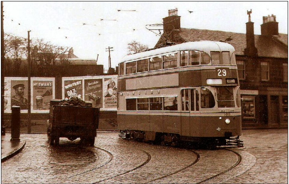
Newly overhauled ex-Liverpool “Goddess” tramcar 1015 rounding Allan’s Corner (“the hairpin”) in Barrhead while on test.
